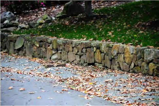
STONE WALL AT GLANDON
