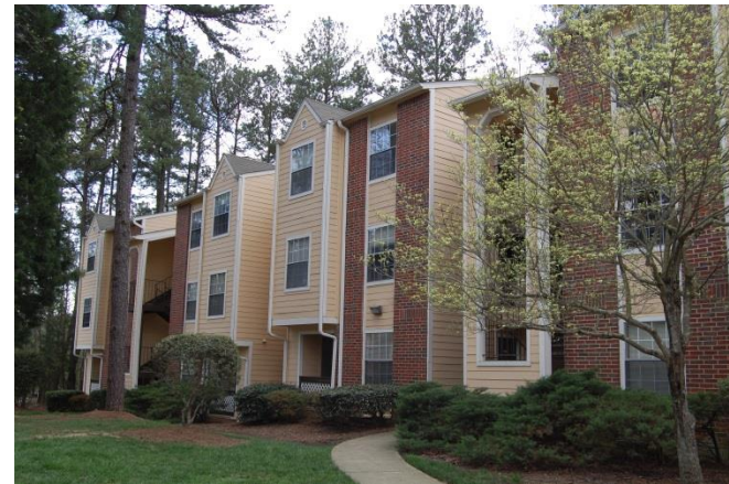
Timber Hollow Apartments
