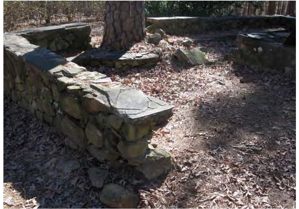
10 Wall at Fireplace
