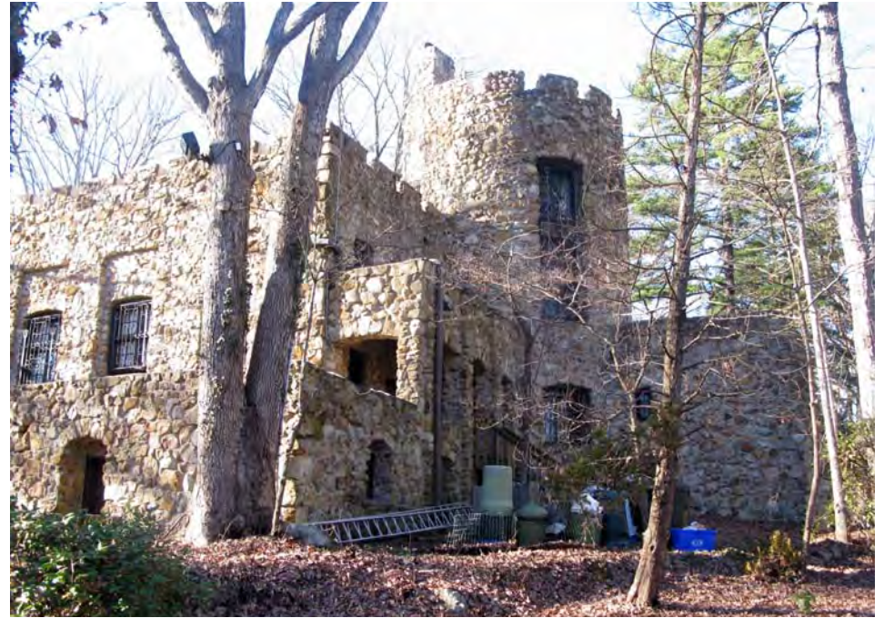
06 South and East Elevations
