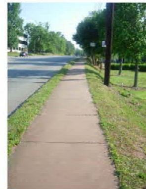
STEEP SIDE SLOPE NEAR UMSTEAD ROAD
