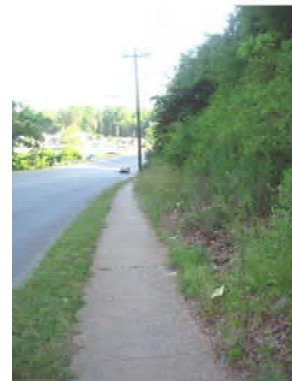
NARROW SIDEWALK NEAR BOLIN CREEK
