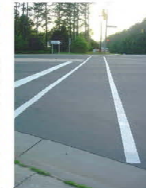
NO PEDESTRIAN REFUGE LOCATED IN CROSSING
