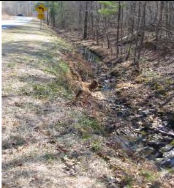
Stream 14A, looking south along Seawell School Road
