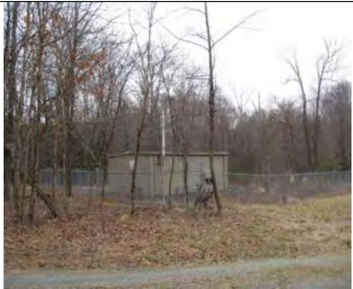
Groundwater Treatment Building, south border
