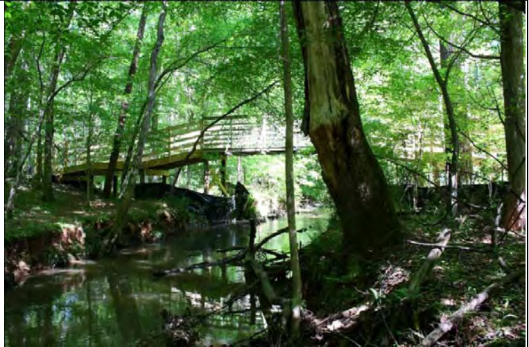
View from Bolin Creek of pedestrian bridge, downstream of the Castlebury mill site
