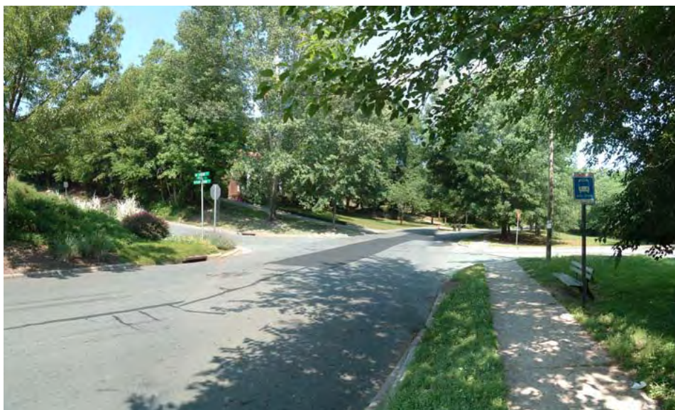
Figure 3.1: Existing Conditions at the intersection of Mitchell Lane and Roberson Street. Proposed improvements will add stop signs and crosswalks at this intersection.
