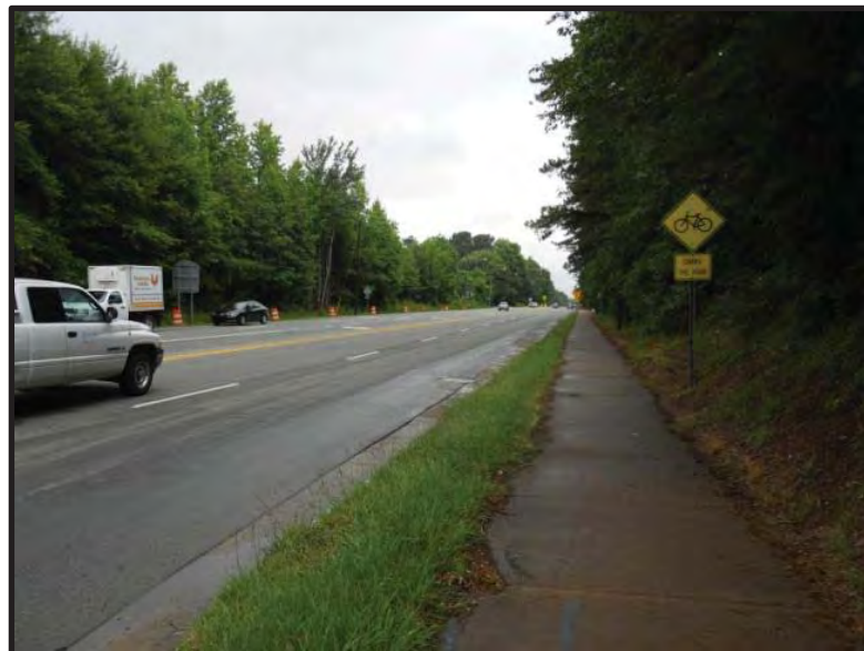
Looking northbound along Martin Luther King, Jr. Boulevard at Estes Drive
