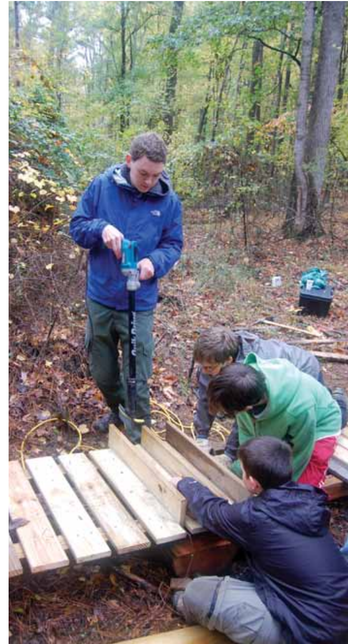
Eagle Scout Boardwalk Project
