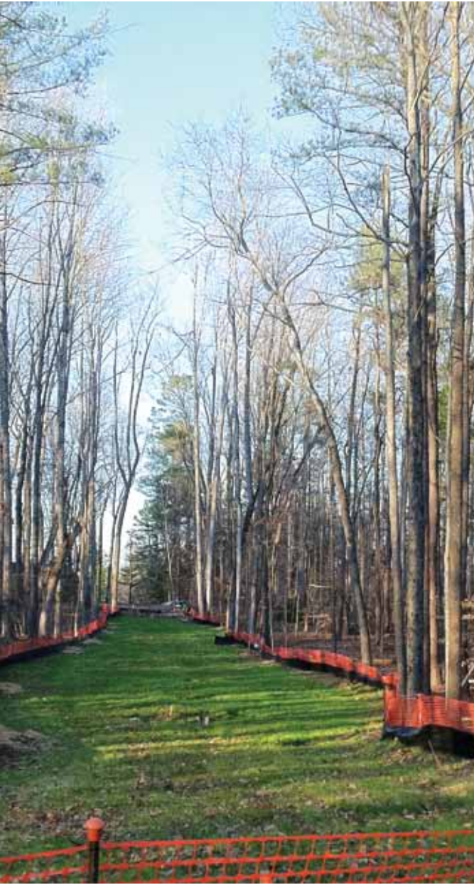
The electric ductbank construction corridor
