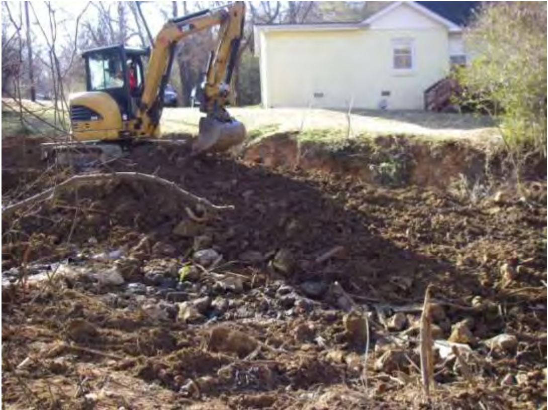
Creating the new channel on the west side
