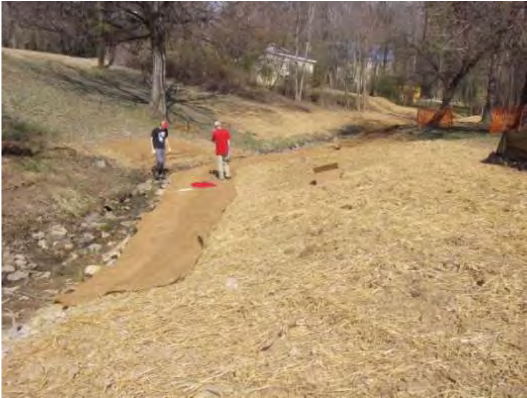
Laying coir matting on the western channel after construction
