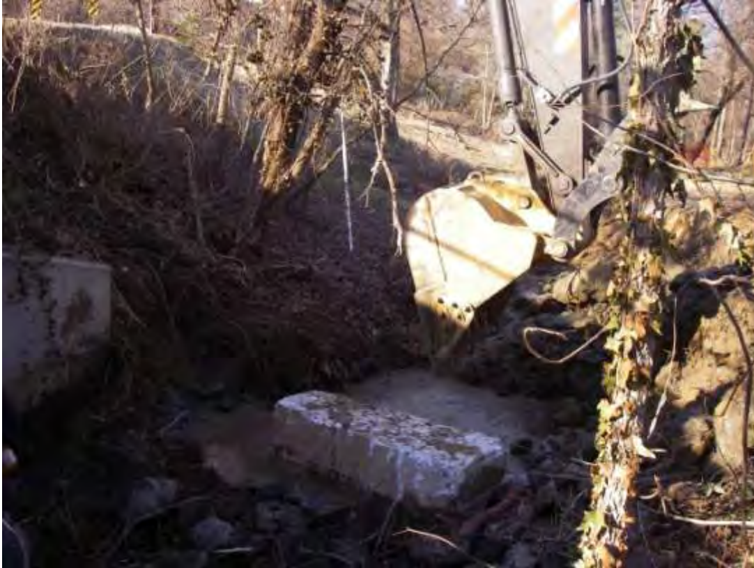
Installing more giant rocks to create step-pools
