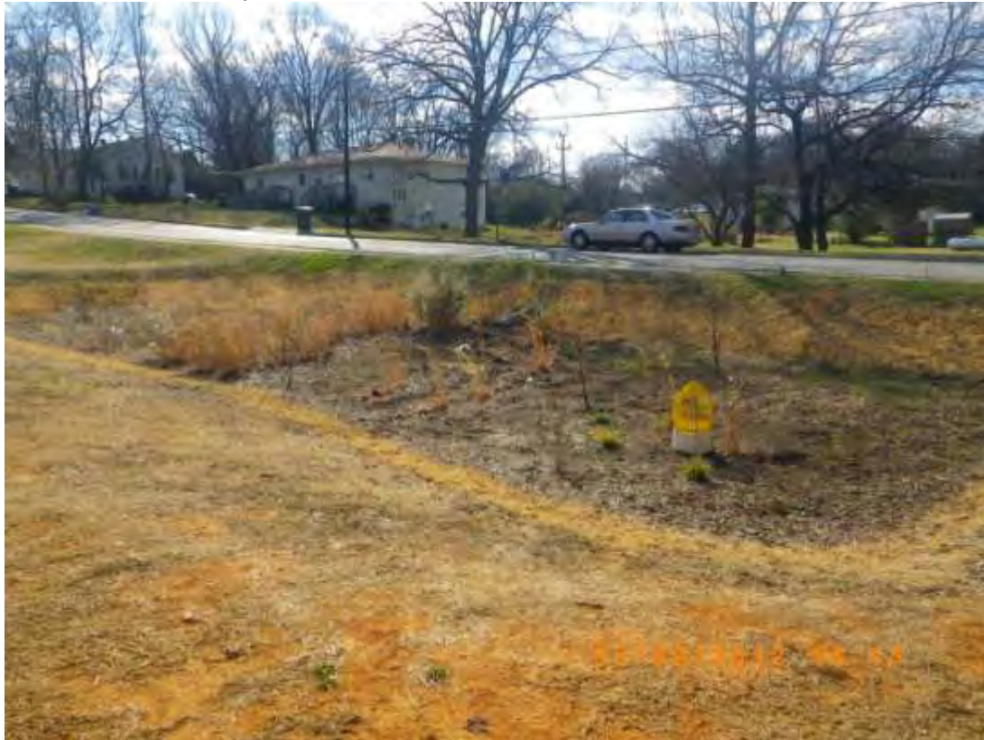
Most of the plants in the bioretention basin have survived the winter and grazing by deer
