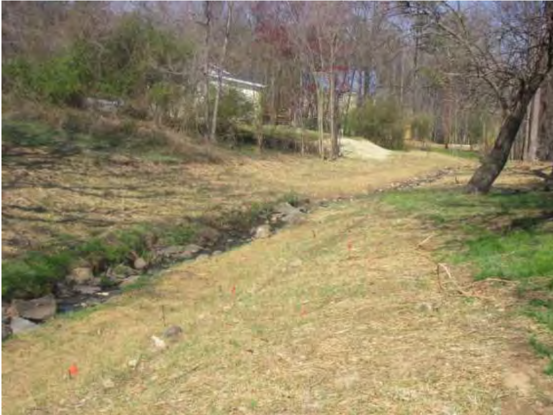
Laying coir matting on the western channel after construction
