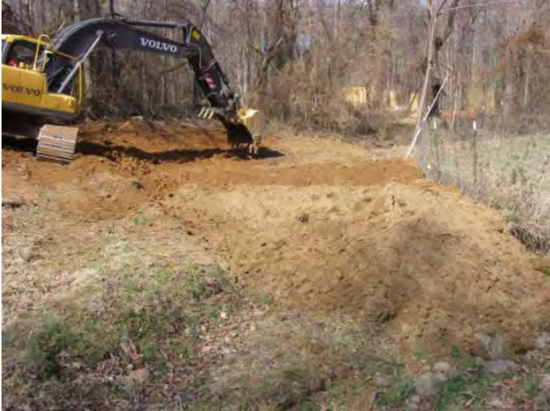
Creating the new channel on the east side
