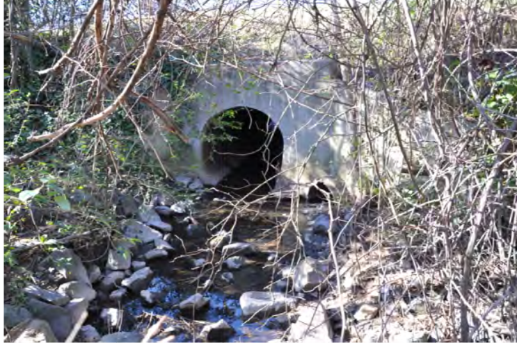
Storm Sewer Outfall
