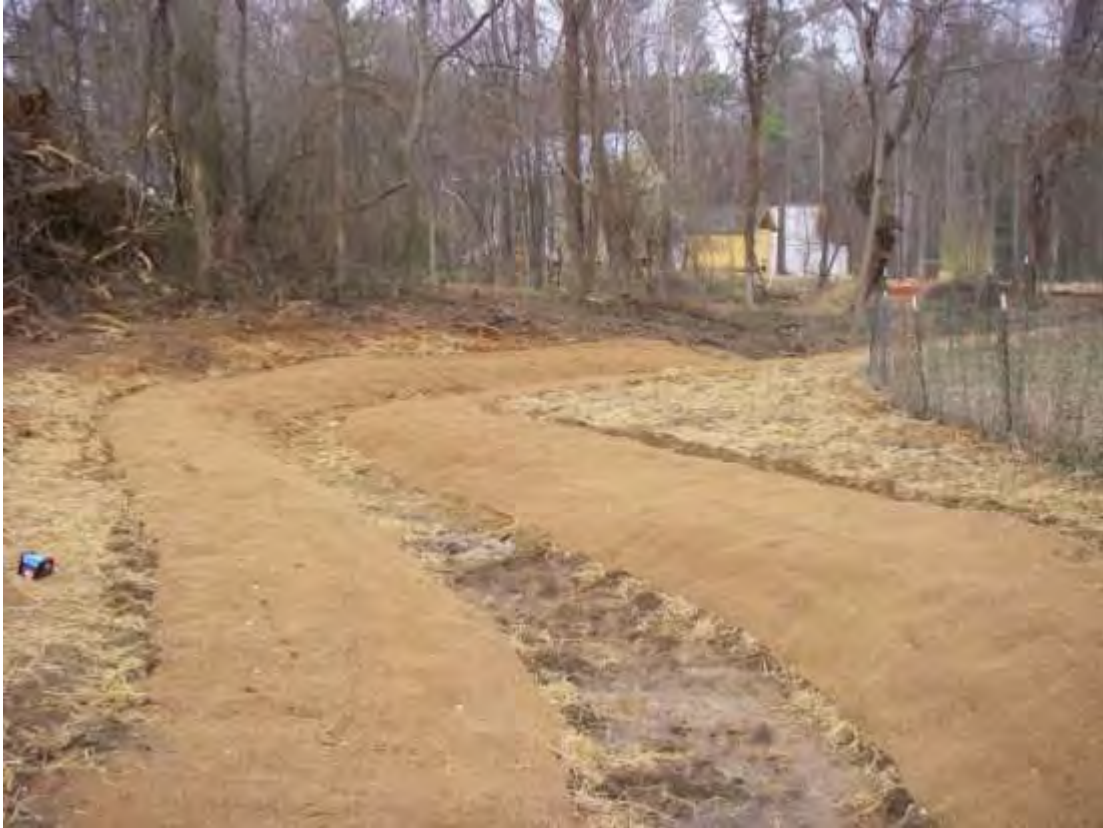
Construction of the eastern channel is complete
