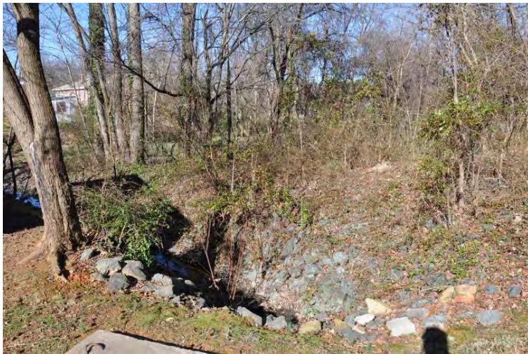
Area 8 View from 30-inch Culvert Outfall
