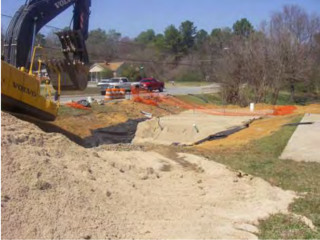
Installing the bioretention basin
