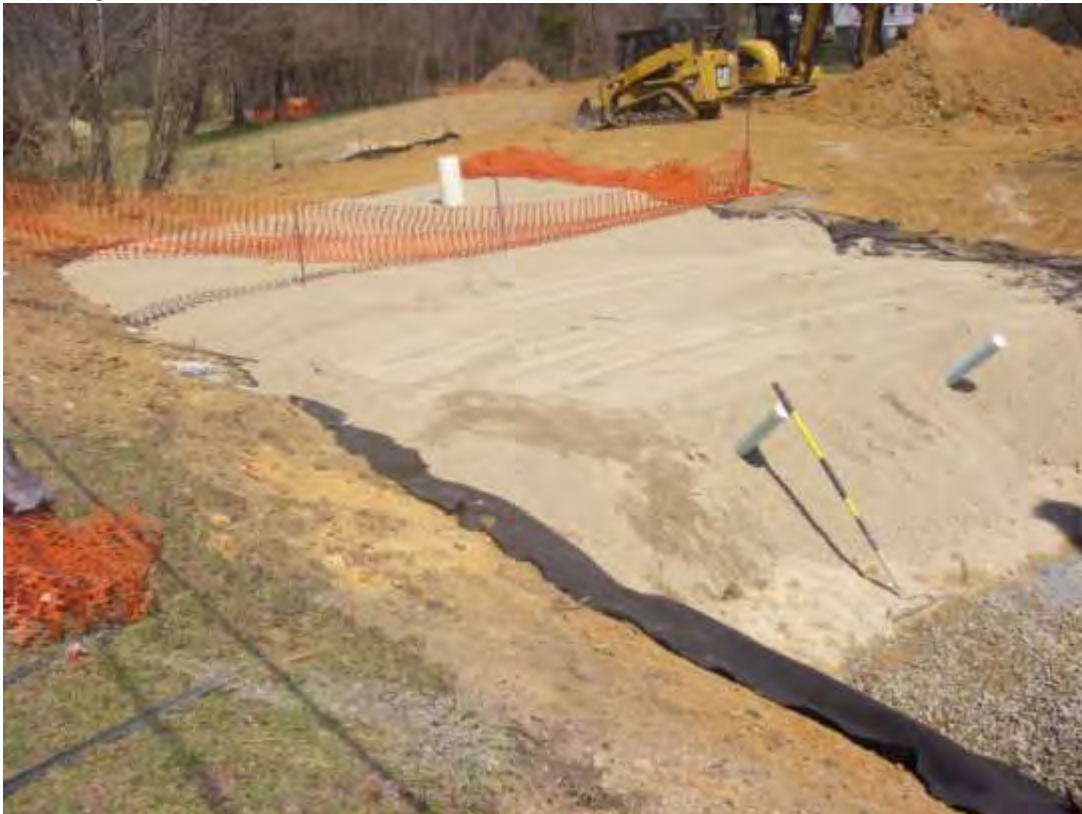
More work on the bioretention basin
