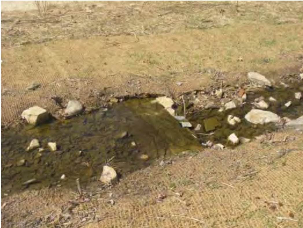
Close-up of a step-pool – there is a giant rock under there, but you can see only about 3 feet
