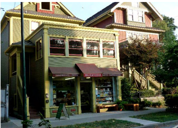
Adaptive re-use helps retain a neighborhood's character.
