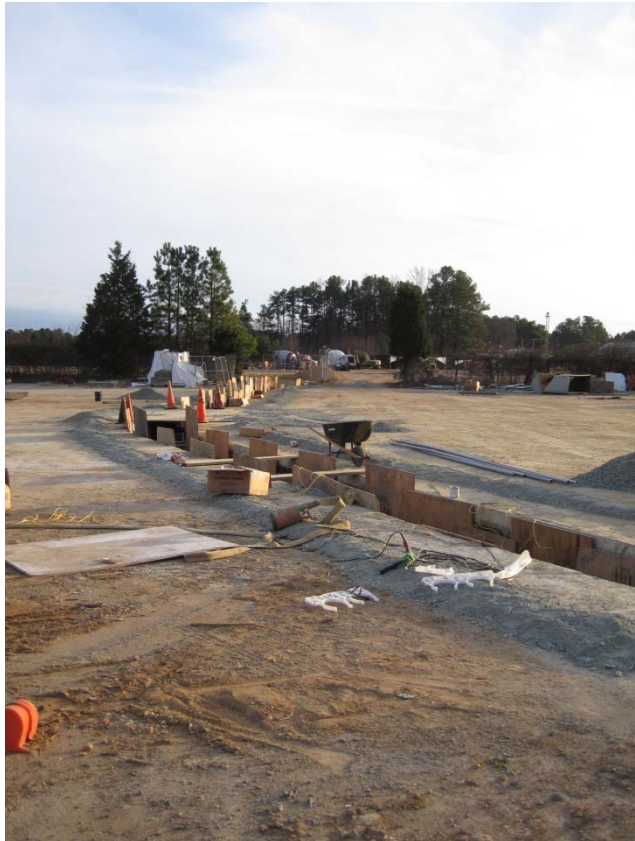
Ductbank installation north of Airport
