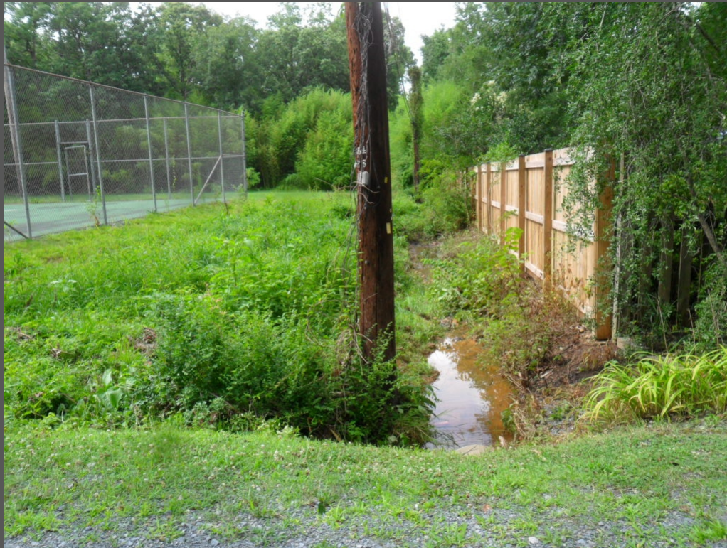
Storm water near Oakwood Park Tennis Court
