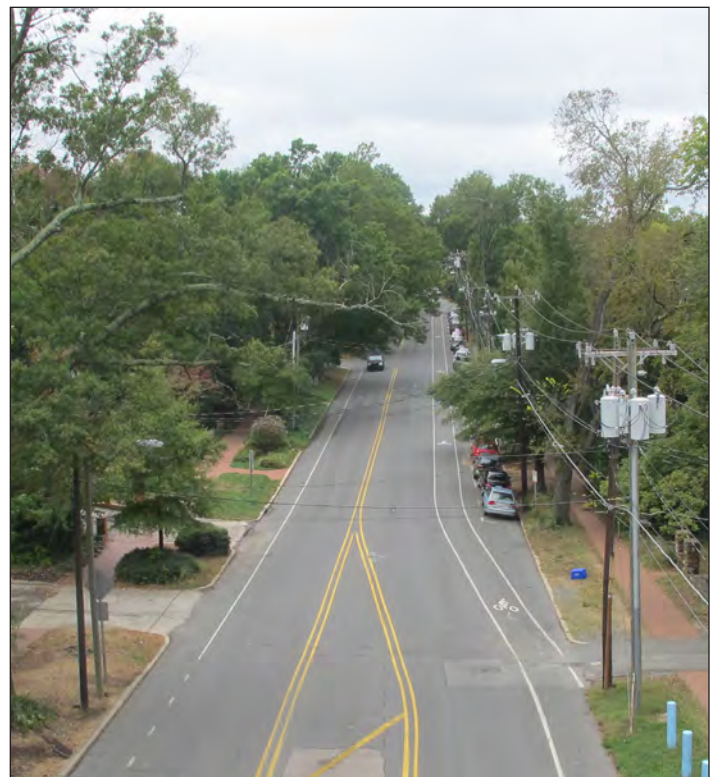
ABOVE: Currently, the on-street parking lane is 10’ wide, the bike lanes are 5’ wide, and the motor vehicle travel lanes are 13’ wide.
