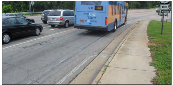
ABOVE: The pavement markings used to delineate this bike lane on the James Taylor Bridge, which have deteriorated over time, need to be replaced
