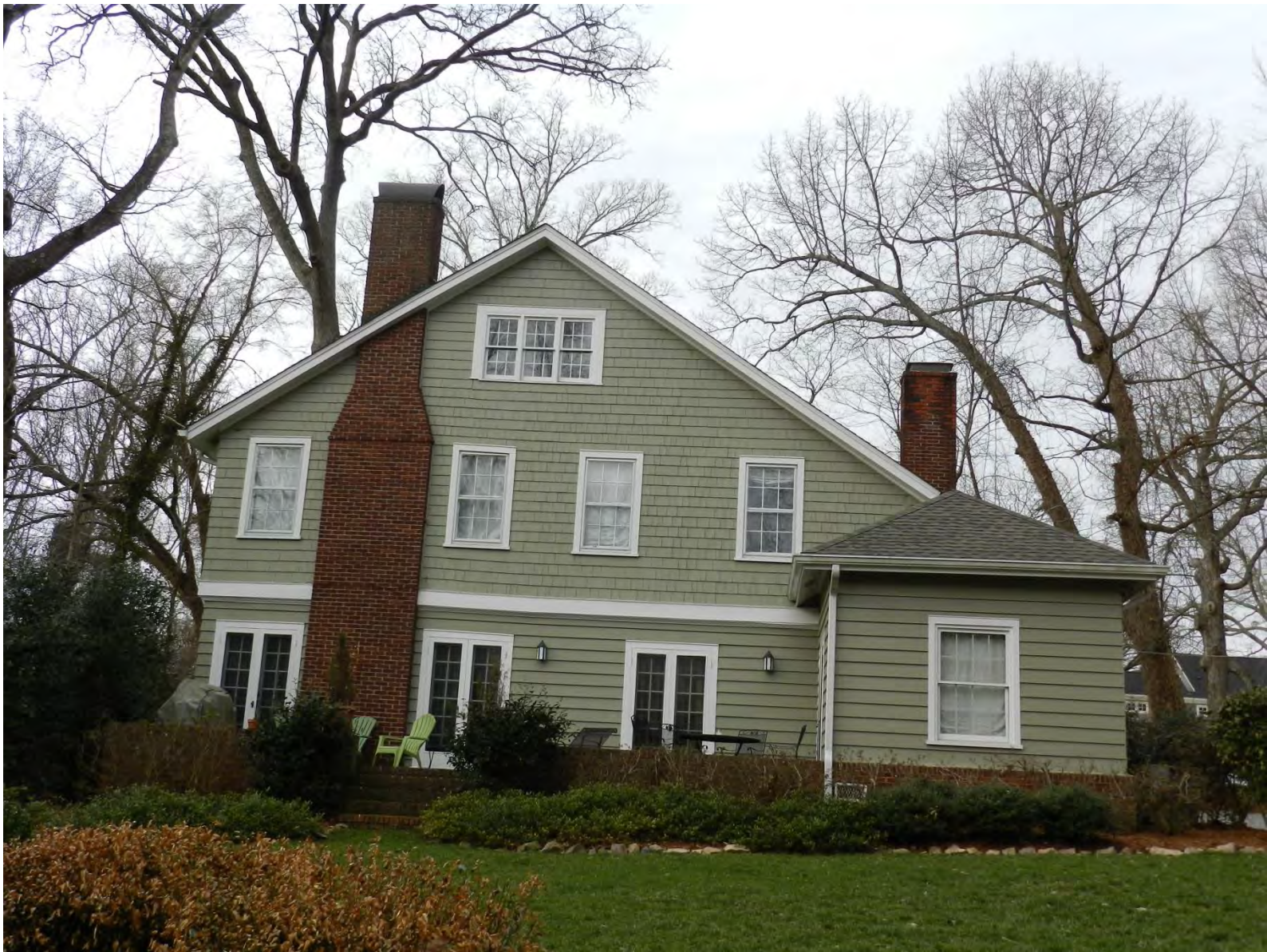
Existing Conditions Photographs Existing East Side Elevation
