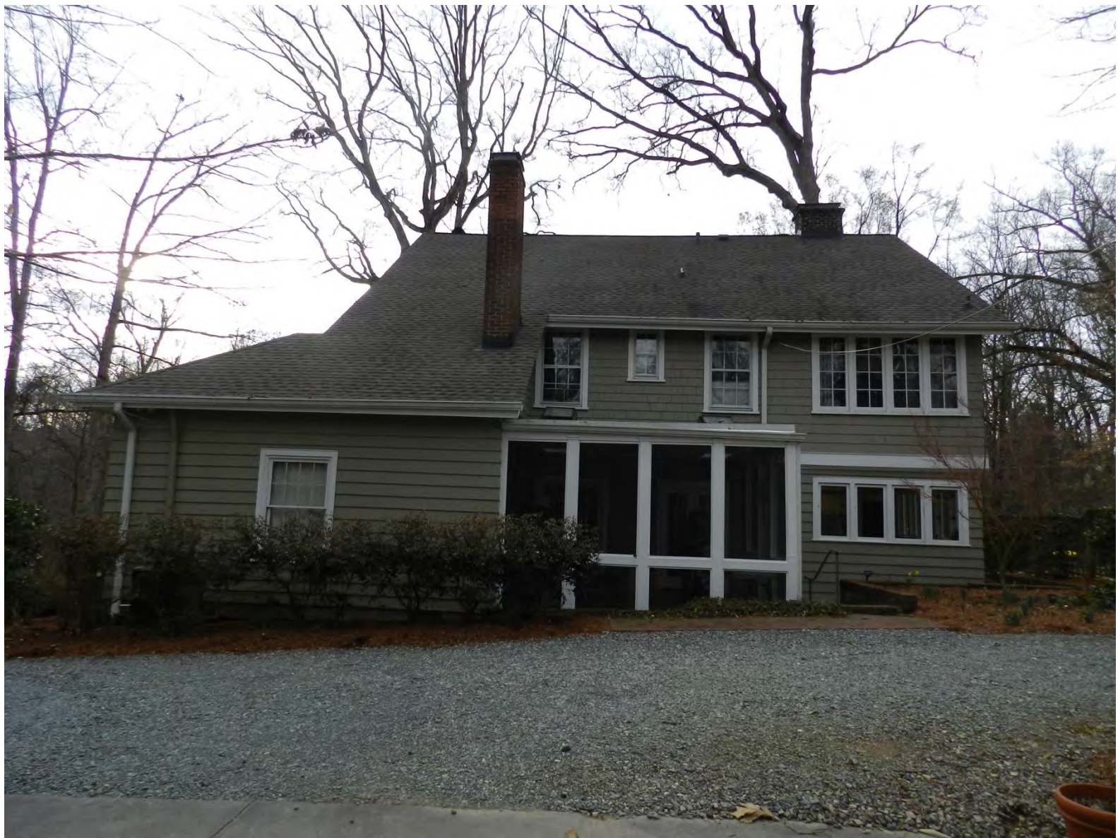
Existing Conditions Photographs Existing North (Rear) Elevation
