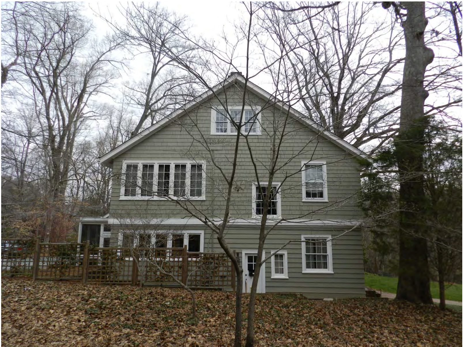
Existing Conditions Photographs Existing West Side Elevation
