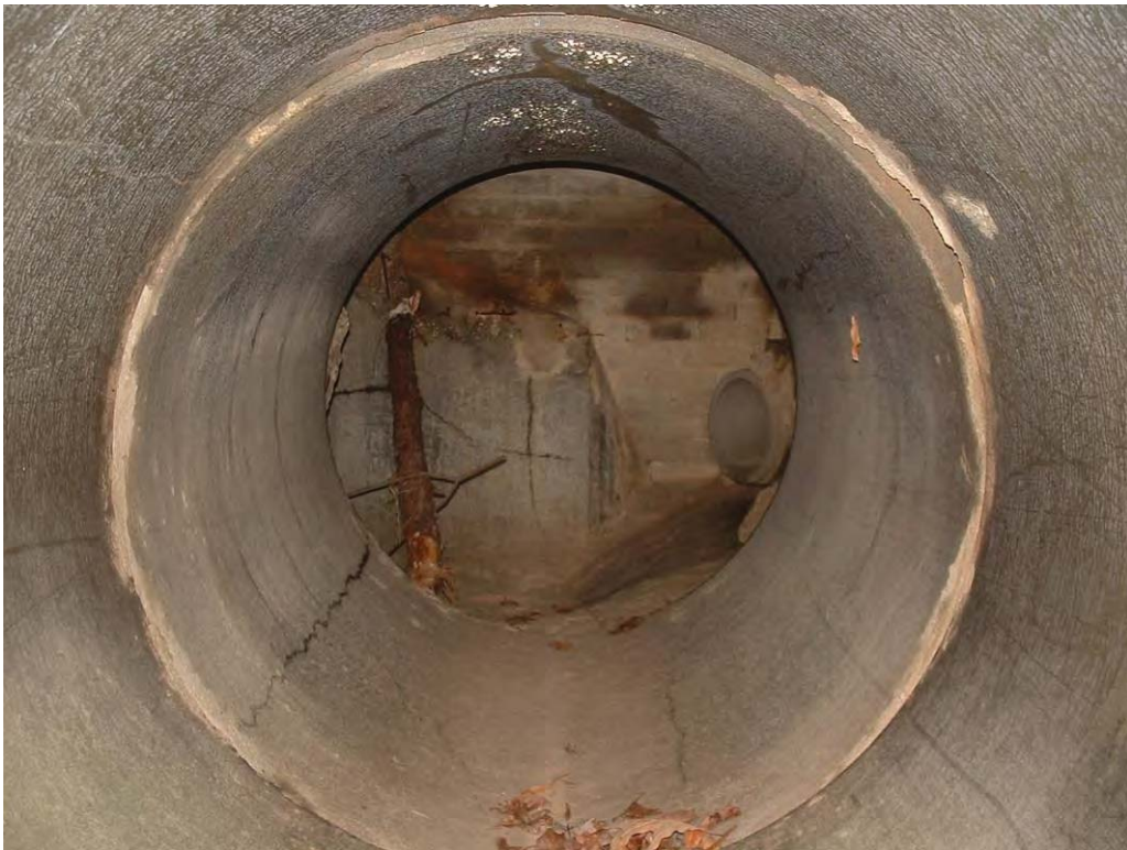
Exhibit C-10. Photos of Tributary 8 Culverts at Ephesus Church Road
