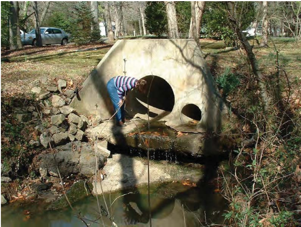
Perched outlet for culvert under LeClair Street
