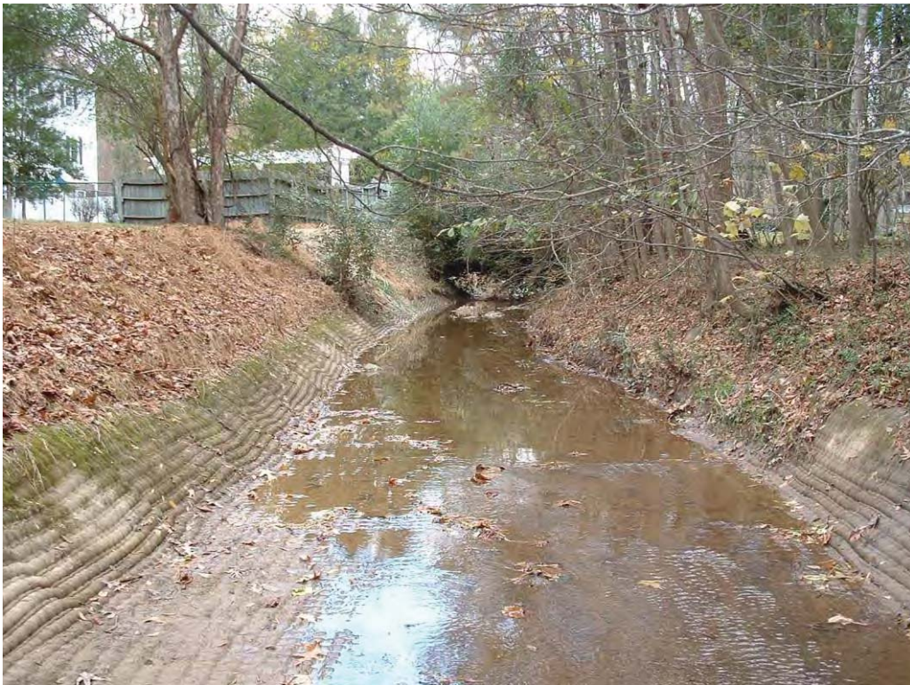
looking upstream from downstream end of concrete lined reach
