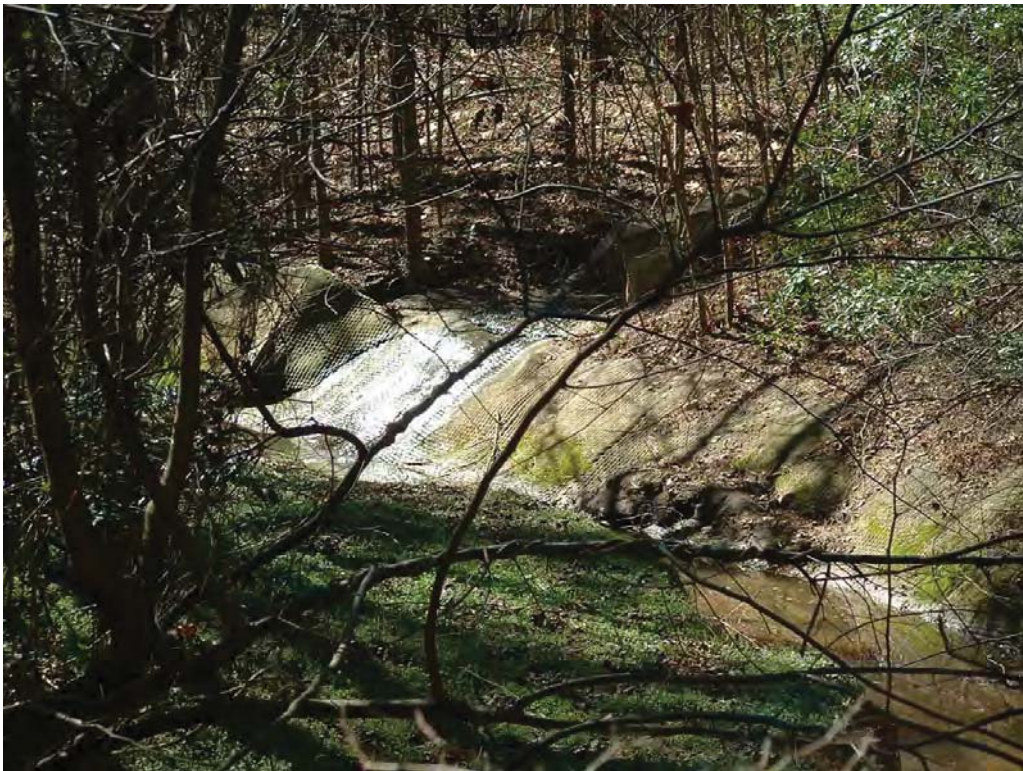
discharge from Tributary 8 into Tracy Branch (prior to concrete failure)
