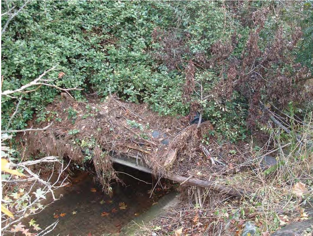
aerial crossing on Reach B
