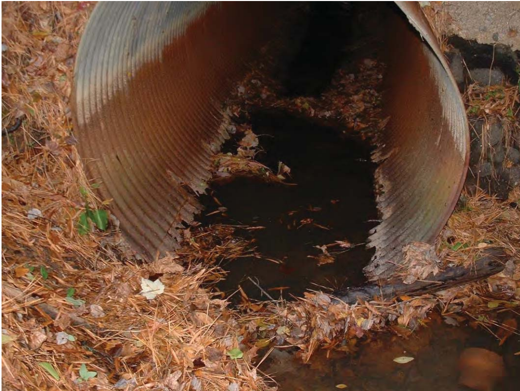
Exhibit C-7. Photos of Colony Lake Outlet and Replaced Fountain Ridge Culvert
