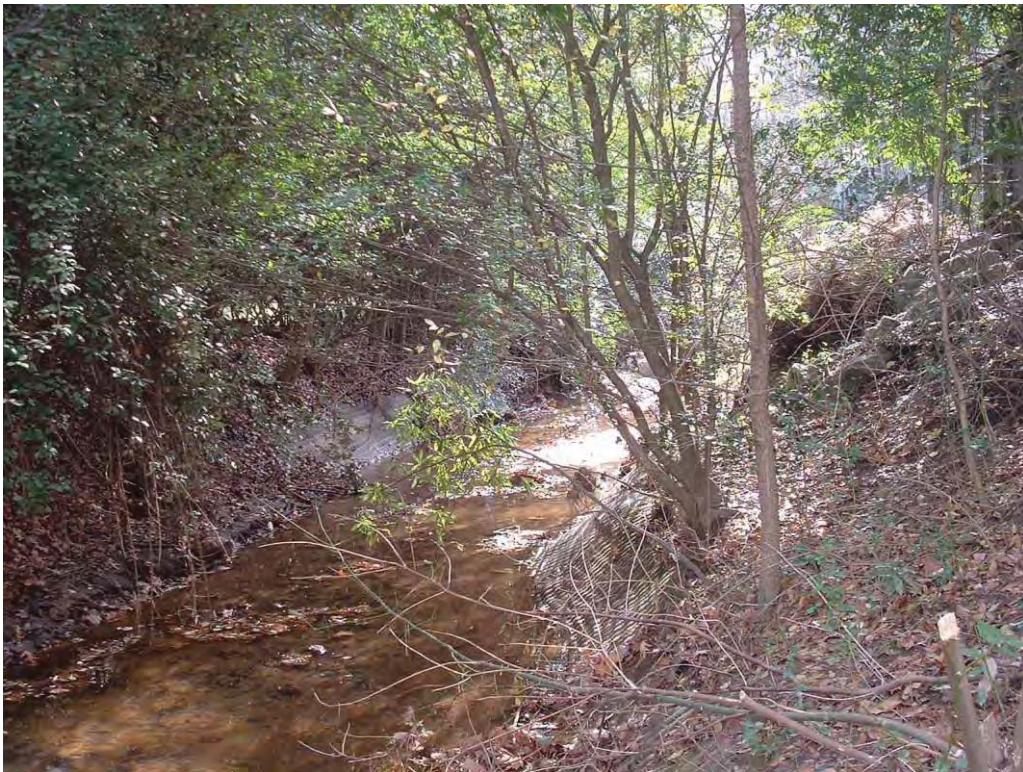
Exhibit C-4. Photos of Reach B Concrete Lined Channel
