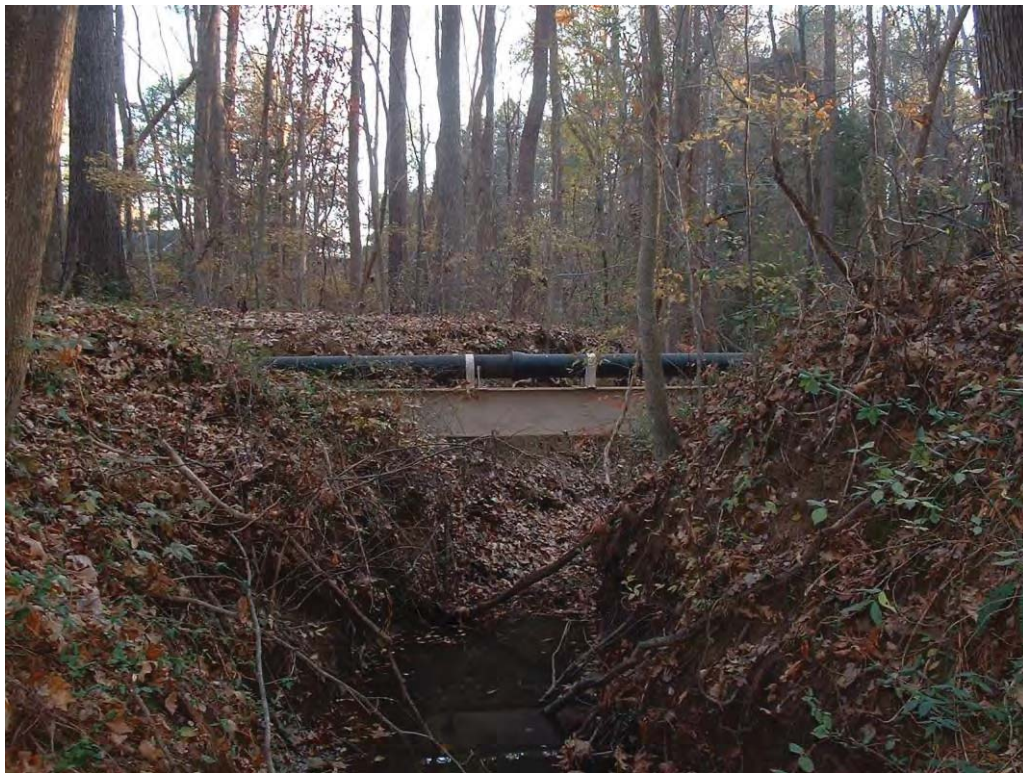
aerial crossing on Reach C
