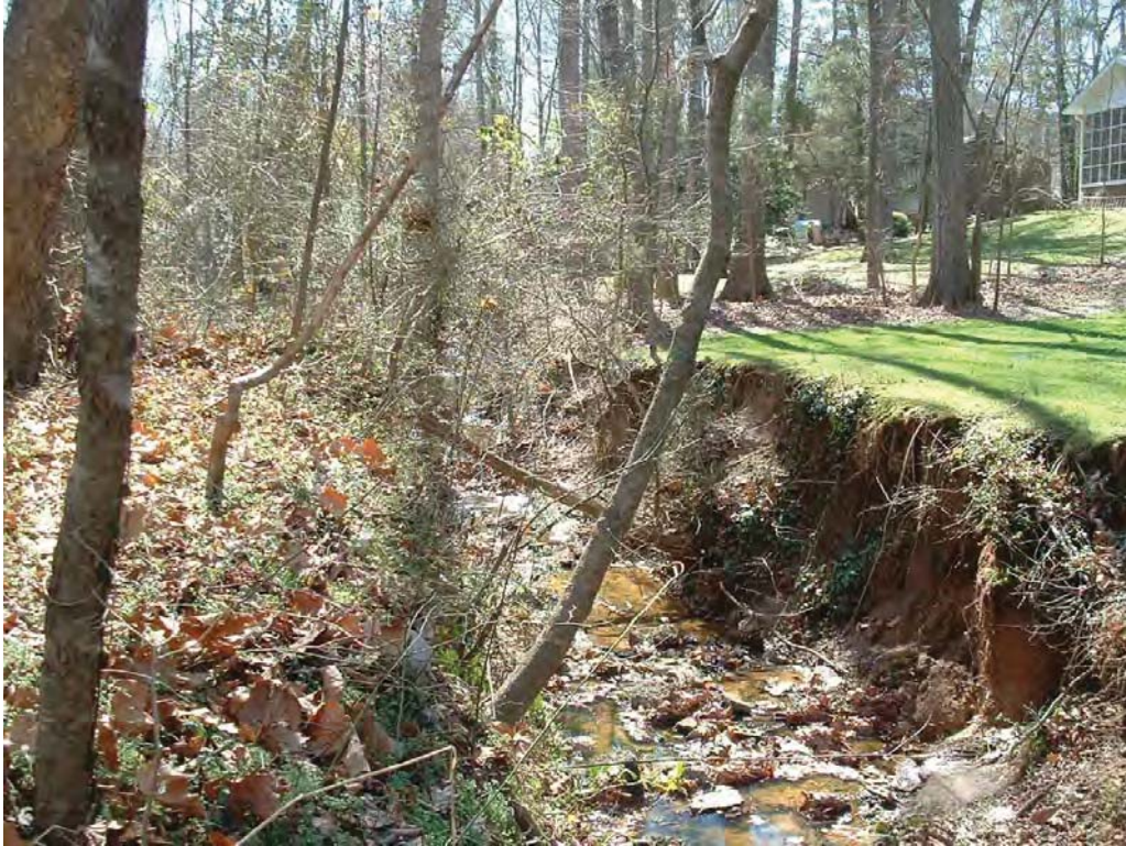
Erosion on Tributary 3; Looking downstream from culvert outlet
