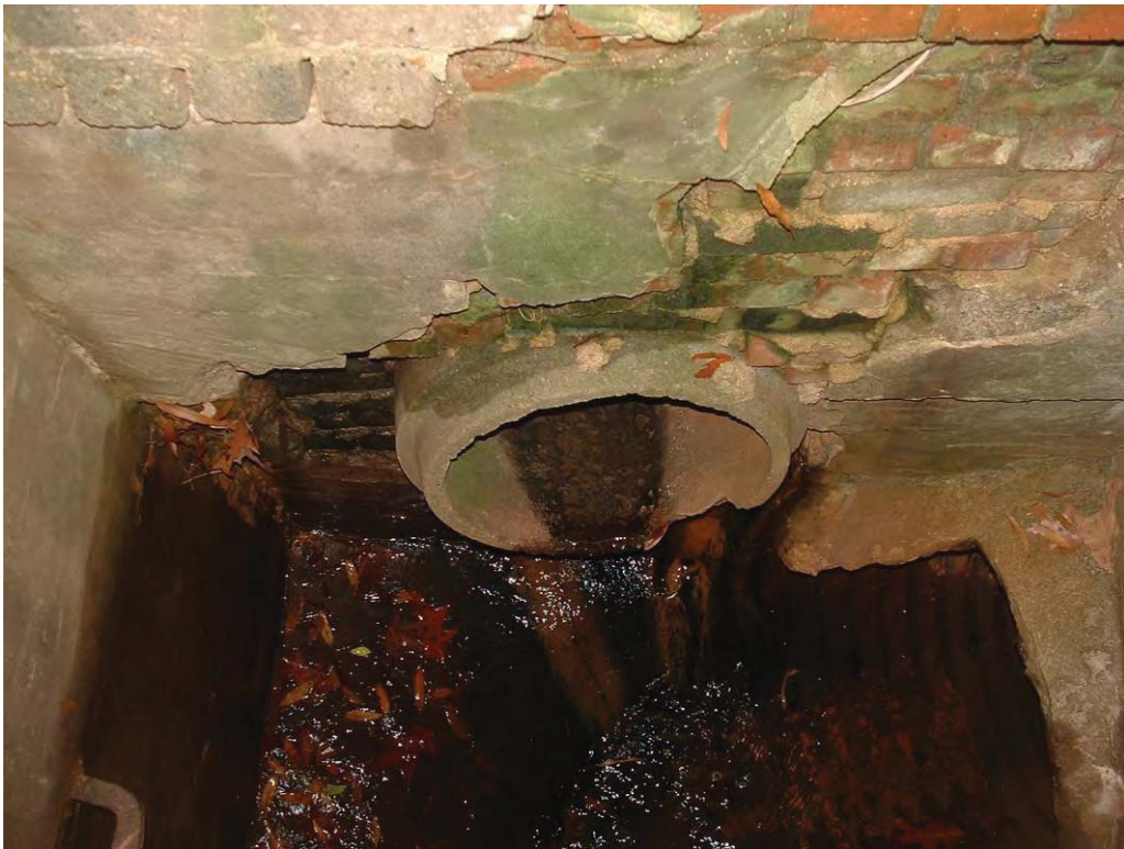
Exhibit C-11. Photos of Tributary 8 Low Flow Culvert at Ephesus Church Rd
