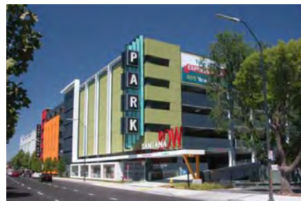
Parking Garage Canopy
