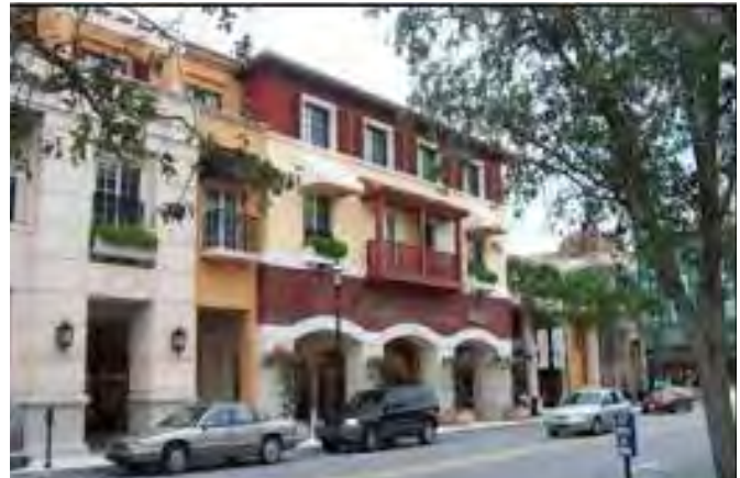
Building projection acting as entrance canopy
