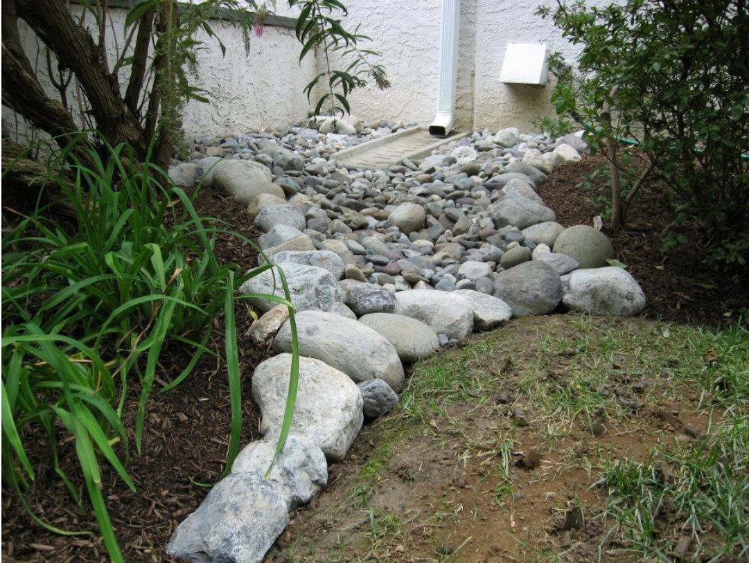
Figure 4.6 – Decorative Residential Splash Block / Energy Dissipater Examples
