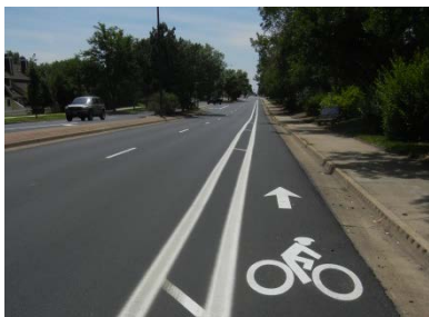
Buffered bike lane with 10 foot travel lanes on 45 mph arterial on Shields Street in Fort Collins, CO
