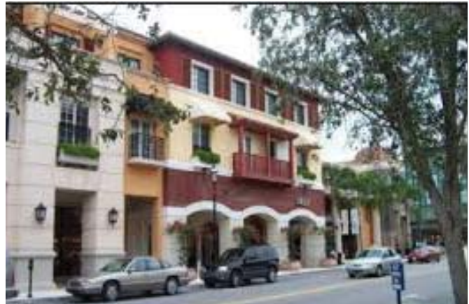
Building projection acting as entrance canopy
