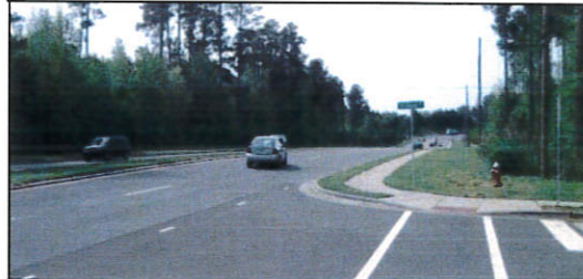
Obey Creek Site Parcel Looking South Near Southern Village P&R Driveway
