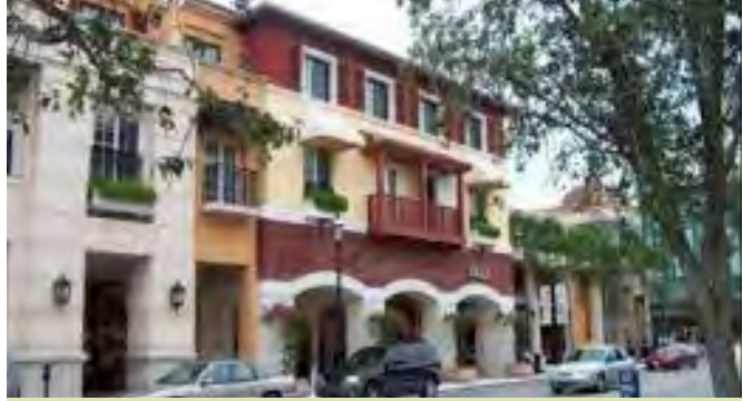
Building projection acting as entrance canopy
