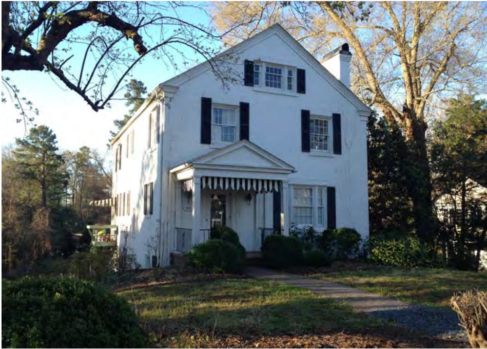
4 North (Street) Side
