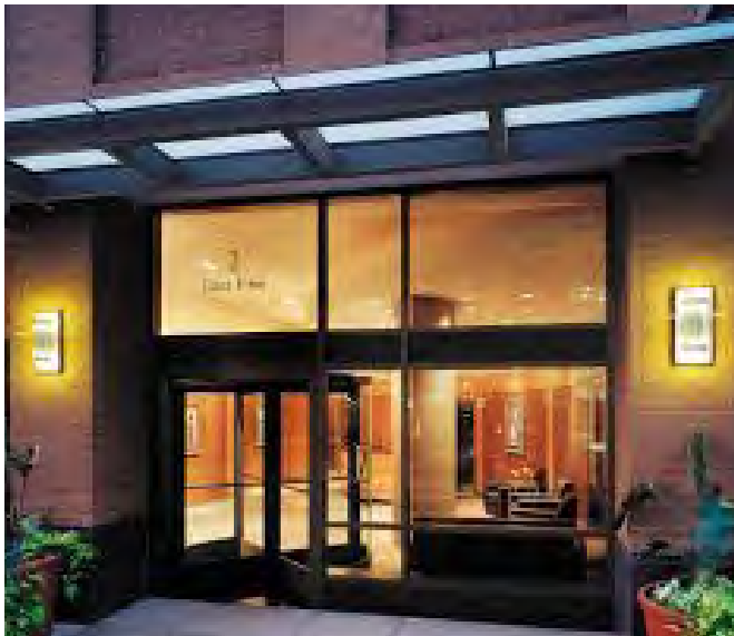
Canopies and recessed entryways protect entries
