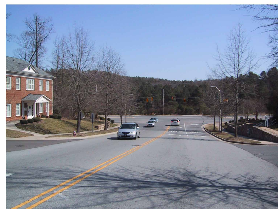
6 - Looking East Through 15/501 From Southern Village Village Entrance
