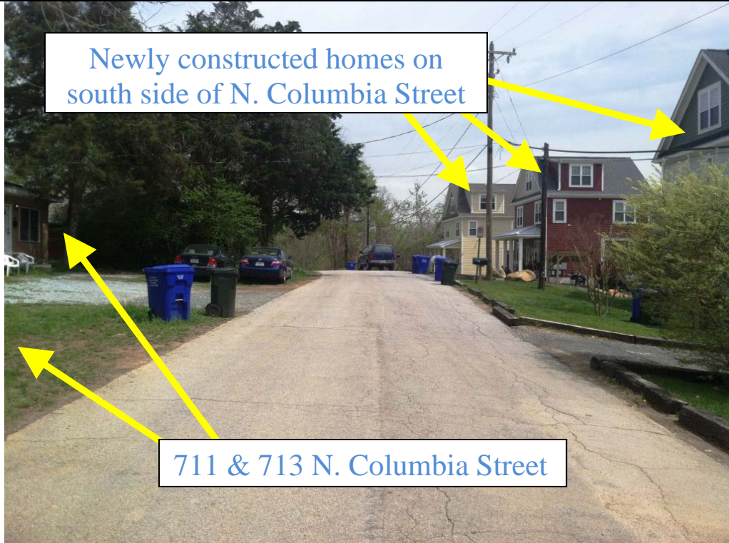
003 Existing Conditions on N. Columbia Street
