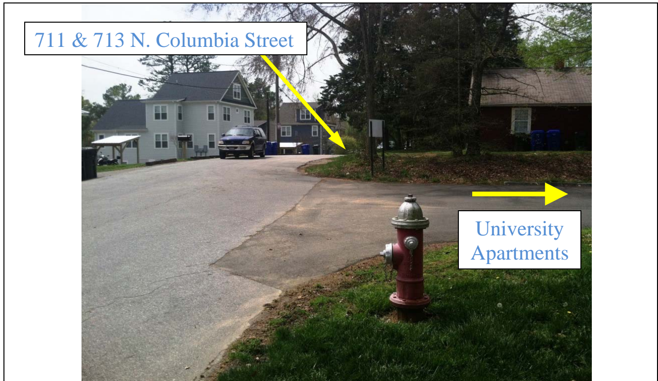
001 Existing fire hydrant approximately 250 linear feet to northeast of 711 & 713
