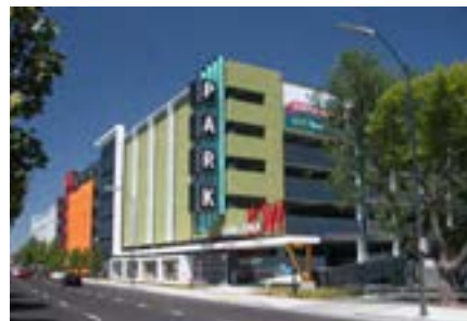
Parking Garage Canopy
