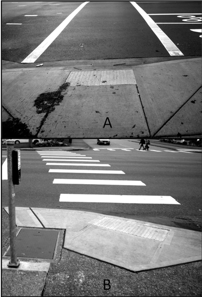
Figure 1. Intersections with perpendicular curb ramps in which (A) the ramp slopes in the direction of travel on the crosswalk and (B) the ramp slopes toward the center of the intersection.
