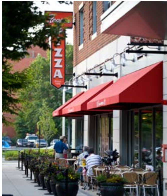
Awnings supported from building wall
