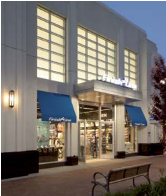
Opaque, ornamental or fritted glass can add visual interest to the upper stories of buildings
