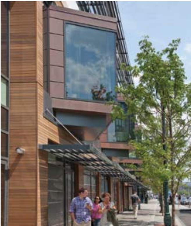
Projecting bays, bris soleil, and varied materials create depth and shadow on buildings
