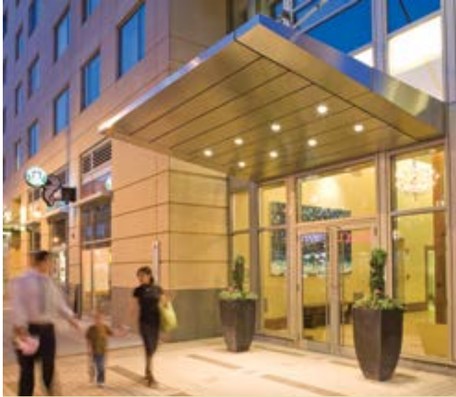
Canopies and recessed entryways protect entries
