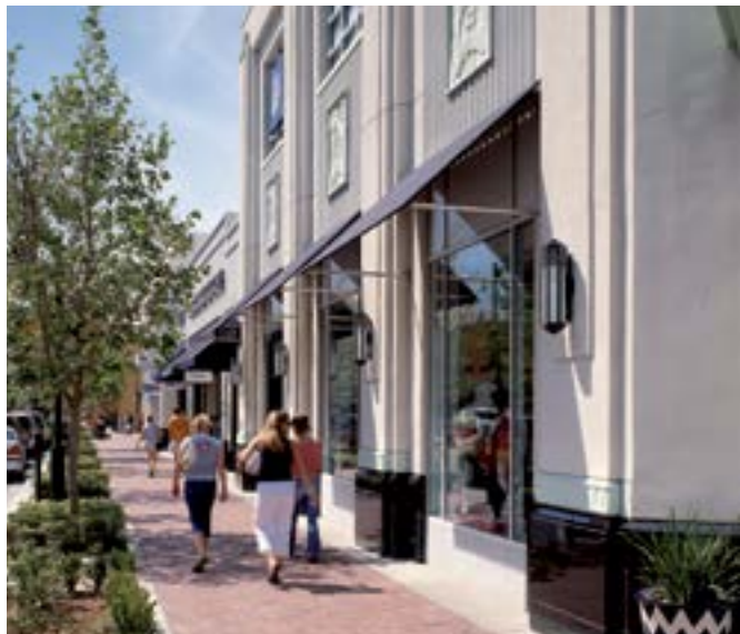
Awnings can provide shade and weather protection
