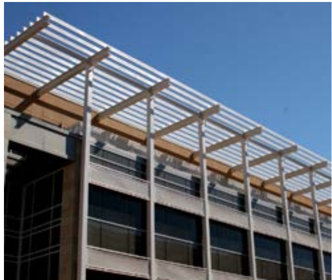
Trellises, cornices, and terraces add human scale to the upper stories of office buildings
