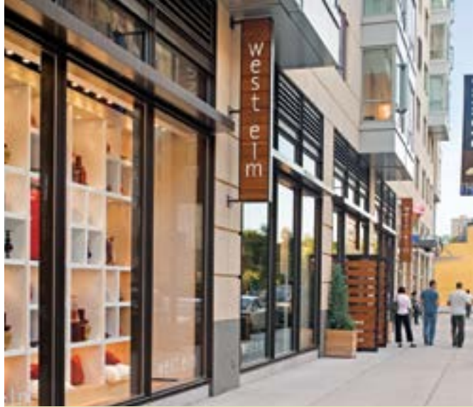
Transparent glass connects exterior space to interior space
