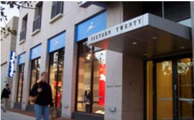
Residential addresses can be integrated into the canopy and the building architecture
