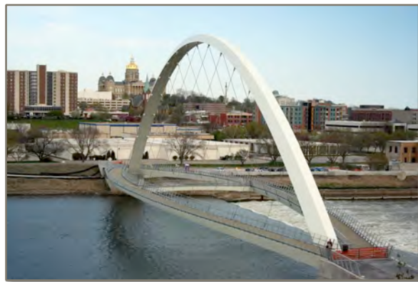
This bridge over the Des Moines River separates directional traffic and uses its structure as an elegant landmark.
