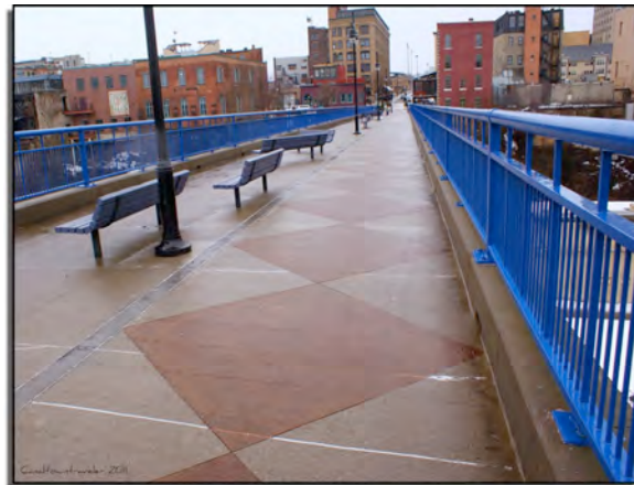
This old rail bed in Rochester, New York was converted to a multi-use pedestrian and bike bridge. Benches along one side of the bridge provide welcome seating to enjoy the views and also serve to subtly remind cyclists to use appropriate speeds.
