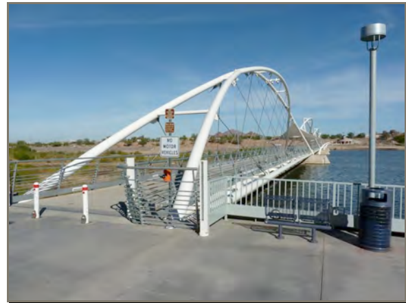
Demand drivers on both sides of this bridge in Tempe were used to ensure widespread use.
