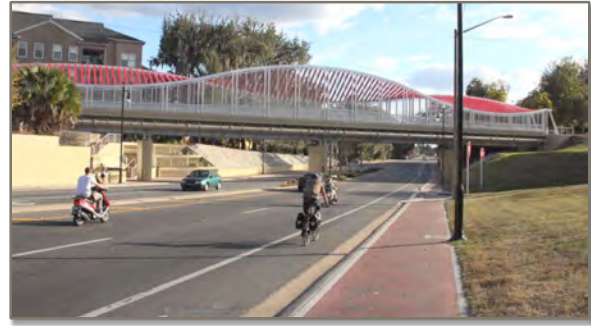
The old bridge enclosure was replaced by this more welcoming structure. The double helix echoes both the rail history and the proximity of the medical center. It also forms the southern gateway to the University.
