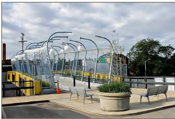
This bridge in Pittsburgh uses an old rail bridge to add sufficient space and greenery to the path. The overhead lights recall nearby factories, and the small open area with benches and planting soften the transition to the parking lot.
