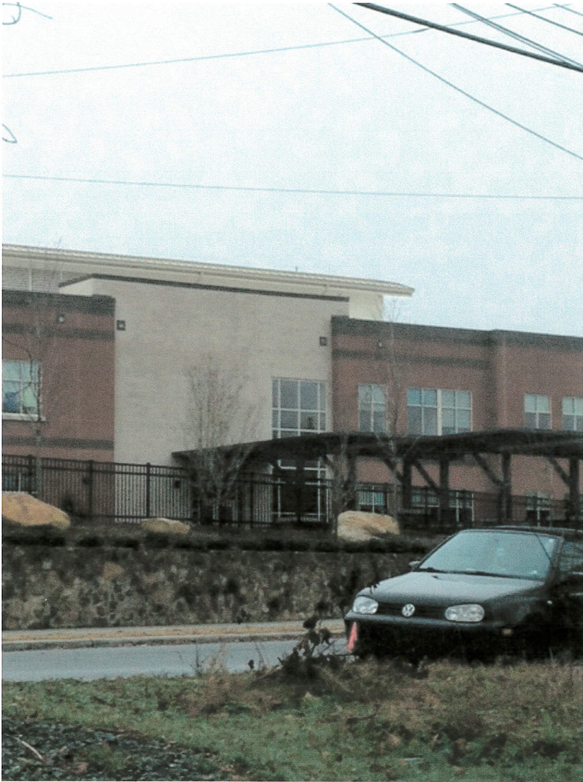
CONTEMPORARY NORTHSIDE SCHOOL ACROSS THE STREET
