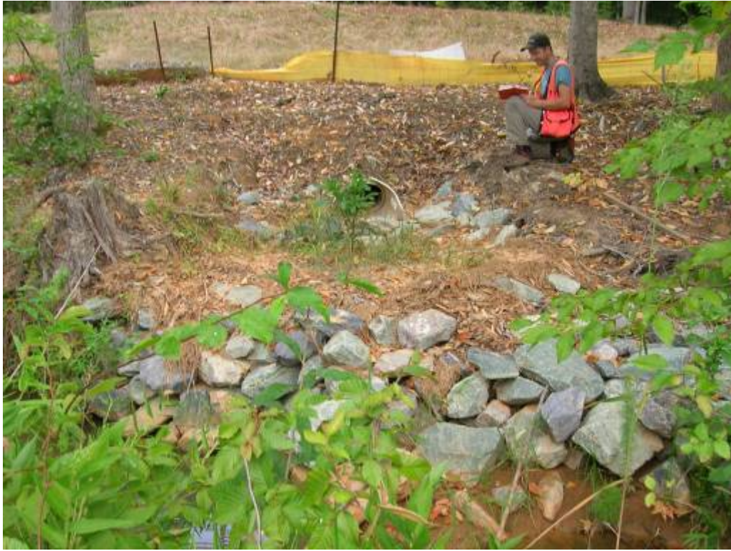
The second sediment basin at Site 6. The pipe outfall is only feet away from the stream, which is located at the bottom of the photo. Facing North.
