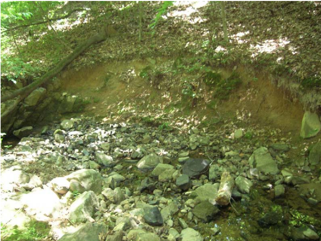
An eroding bank on Cole Springs Branch near Site 25. Facing downstream.
