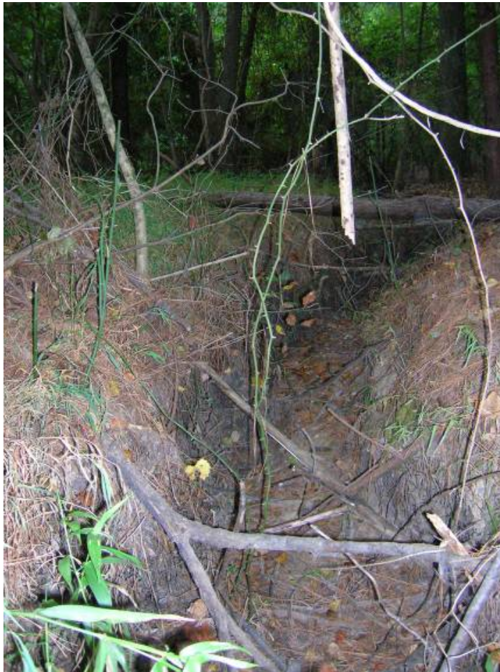
Downstream of the headcut. Facing upstream.
