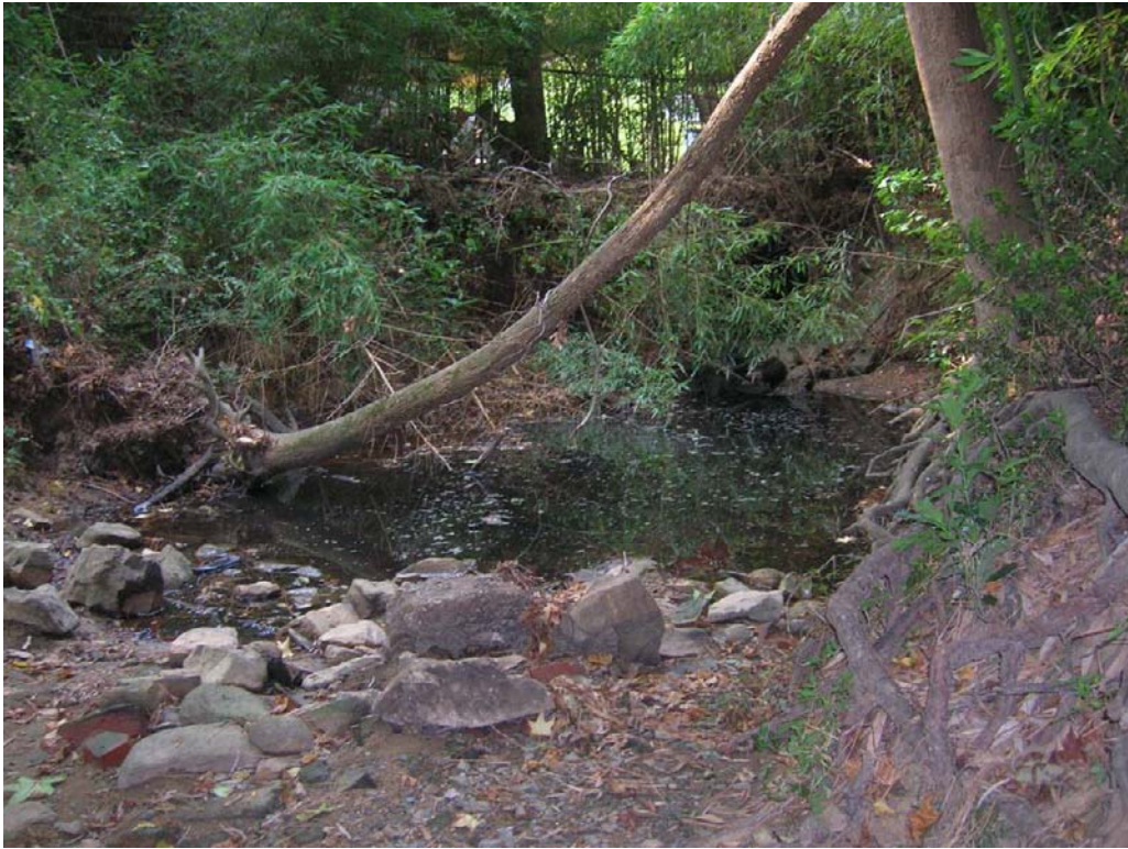
The upstream end of a channelized stream, where a stormwater outfall discharges into a large pool. Facing upstream.
