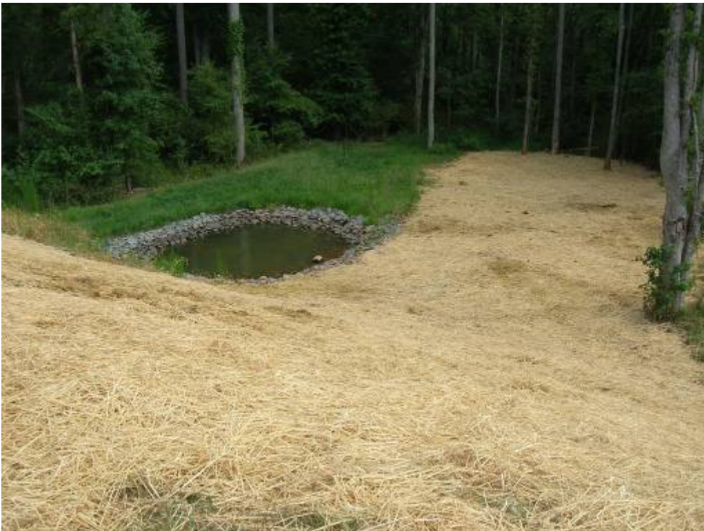
The stormwater basin one month later. The berm has been removed and the site re-seeded with grass.
