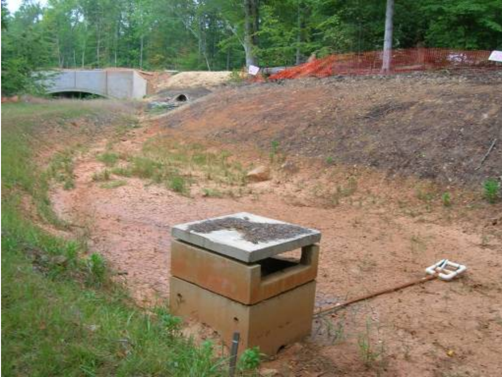
Site 5. The sediment basin outlet structure, facing northwest.
