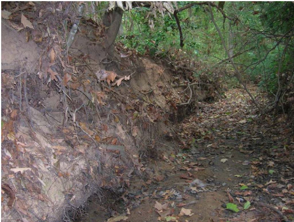
Eroding banks along the stream. Facing downstream.
