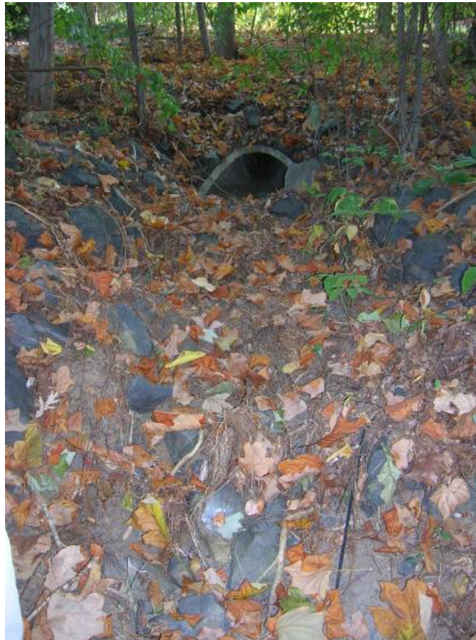
The stormwater outfall pipe below Hotelling Ct. Facing northeast.
