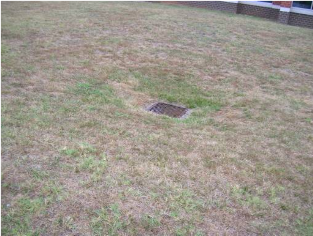
A drop inlet at the middle school. Each of these could be converted into a bioretention area.
