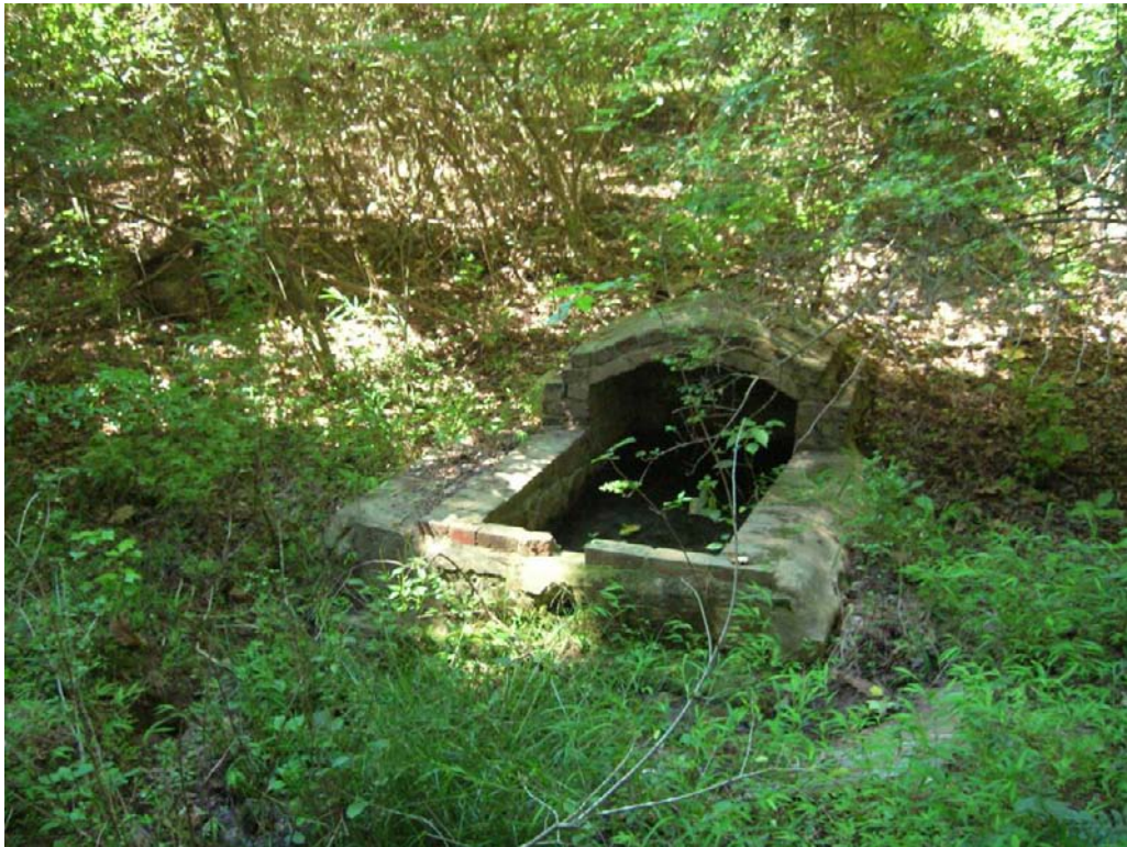
An old spring-head improvement near Site 26.
