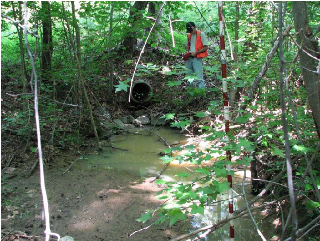
An existing sediment basin below a gravel driveway and culvert. Facing north towards the driveway.
