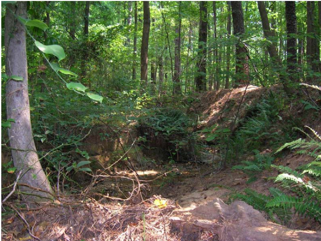
Facing downstream where the ditch from the dissipating structure meets the stream. Note the eroding, partially caused by the flow discharging from the ditch.
