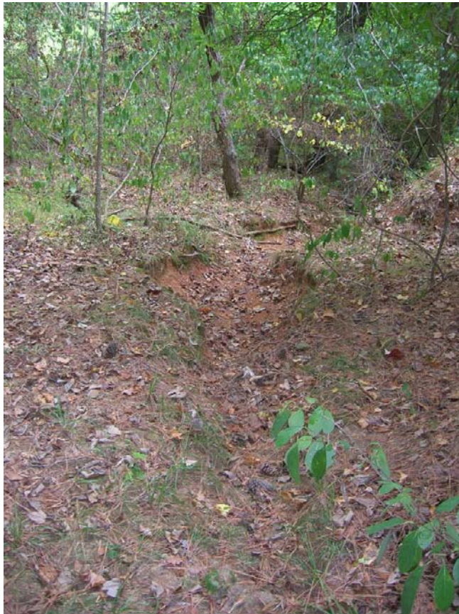
Where the flow has concentrated, an eroding channel and headcut has formed. Facing downstream.
