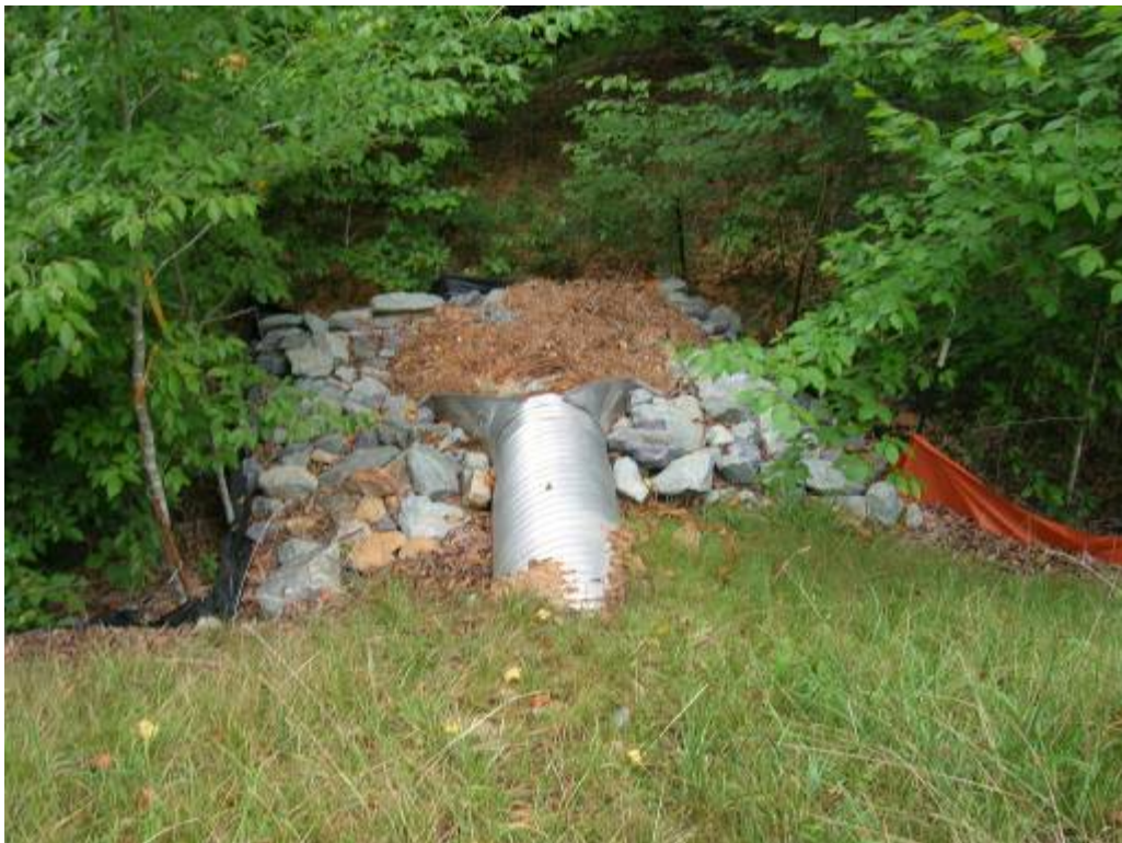
The stormwater outfall of the sediment basin at Site 5. Facing south.
