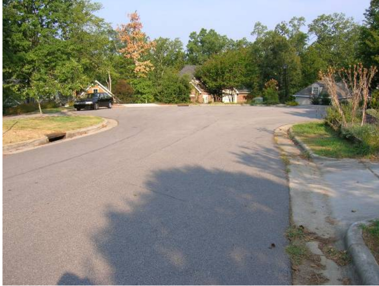
A view of Hotelling Ct, which comprises part of the drainage area of the basin at Site 30. The existing BMP is downhill and to the left of the photo. Facing northwest.
