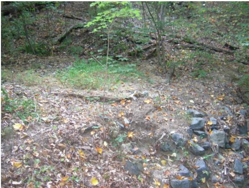
The existing BMP has filled in since its construction. Facing southeast.
