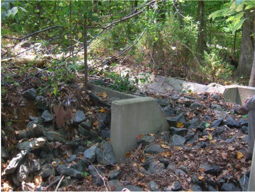
The concrete flow dissipation structure at Site 4.
