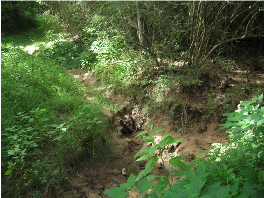
The upstream end of the floodplain ditch, where it is met by stormwater flowing from the nearby road.
