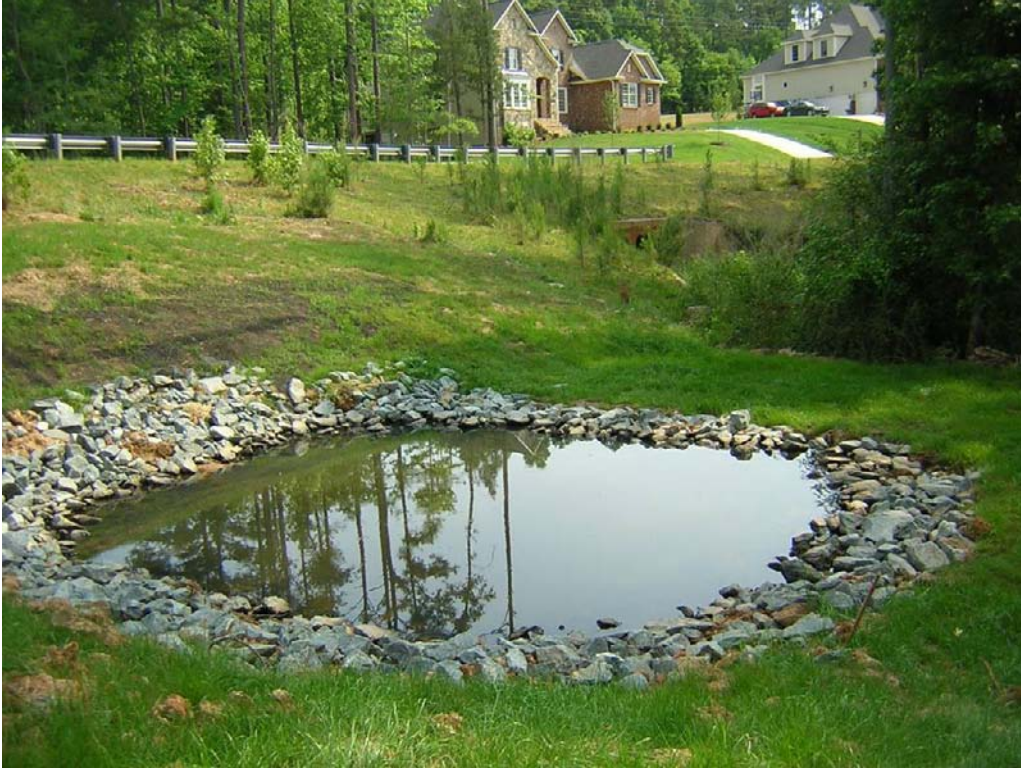
An existing stormwater basin at Site 8. Facing northeast.
