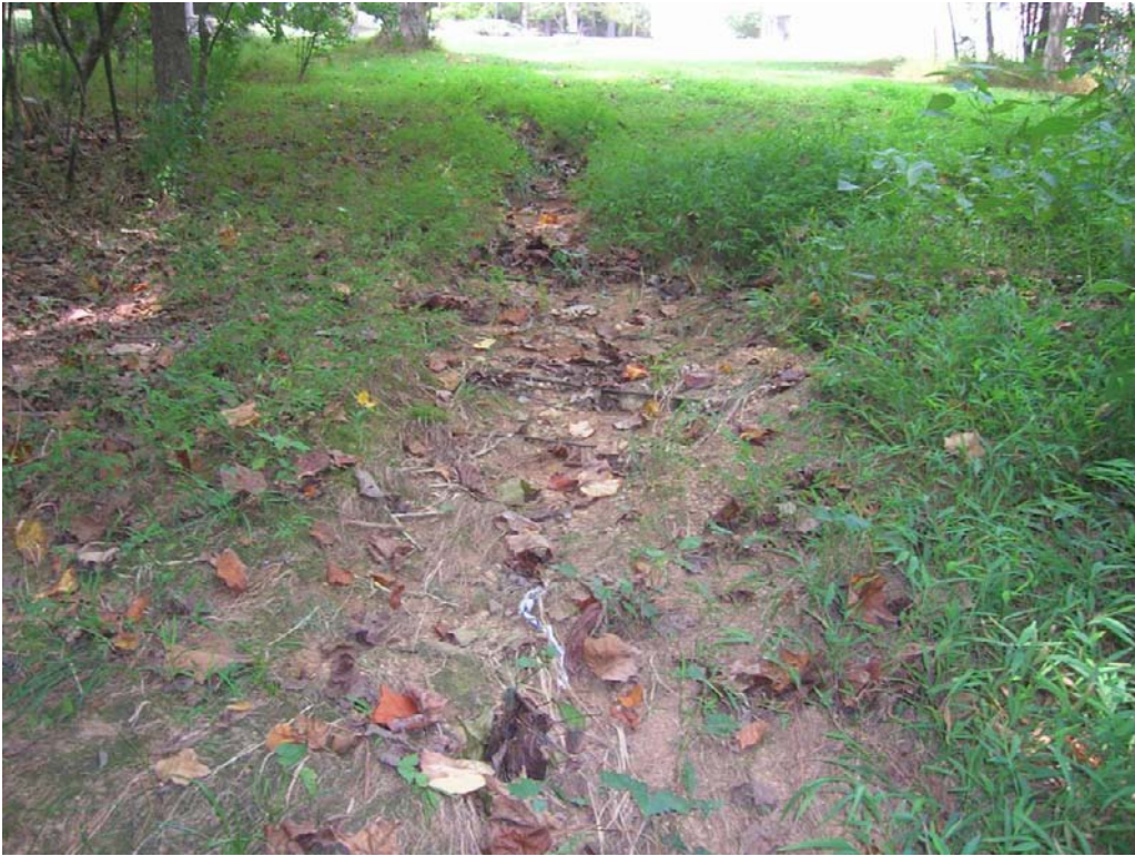
Scour areas are present across from a utility easement, behind the backyard of several houses. Facing west towards the houses.
