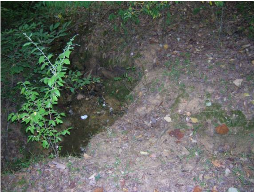
Downstream of the headcut, the channel is much more incised. Facing downstream.
