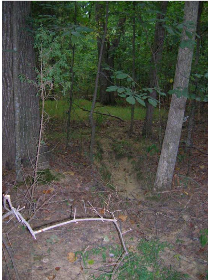
An eroding channel and headcut have formed in the floodplain of Jolly Branch.
