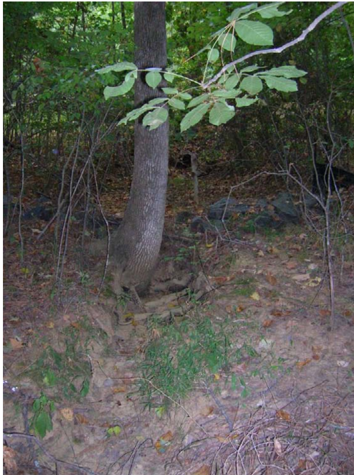
A view of the rip-rap berm around the basin. An eroding channel has formed below the basin. Facing north.
