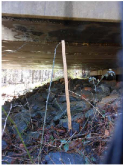
Water in Dec. 30 video was within 39 inches of bottom of bridge (at time video was taken.)
