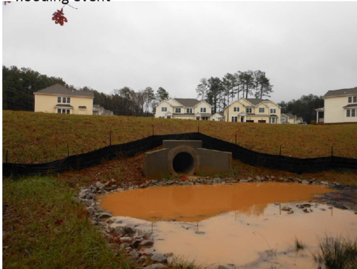
Burch Kove nearing completion - December 30, 2015 flooding event
