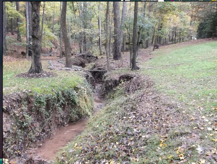
Oxford Hill Rd stream stabilization and buffer enhancement
