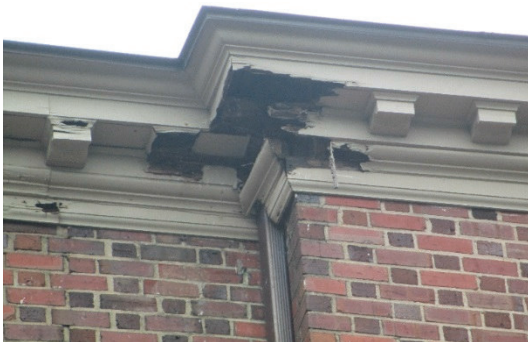
Area below catch basin on west side.
