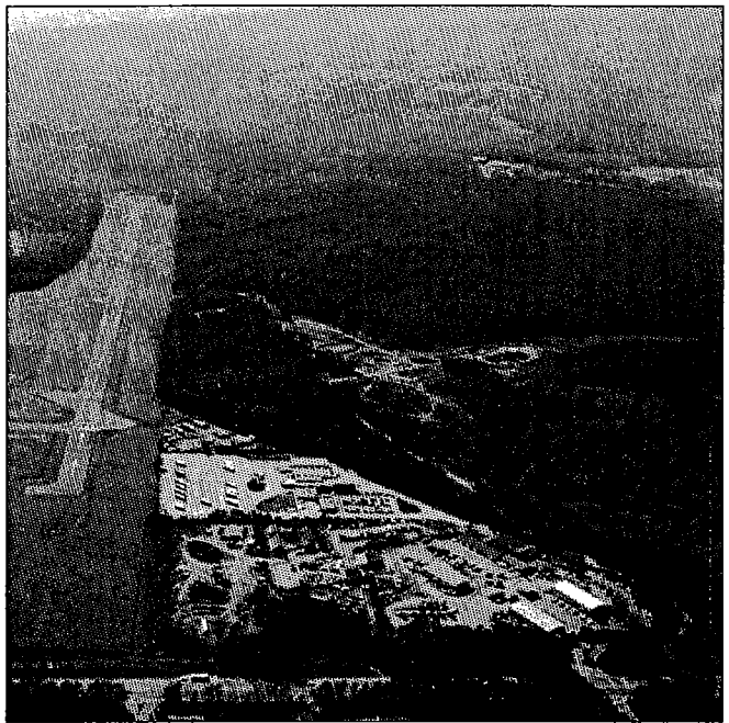
Aerial view of existing Municipal Yard and runway along Airport Road
