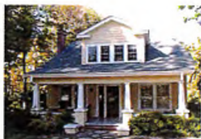
Small Neighborhood Building
