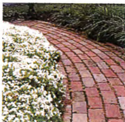
Photo showing pervious paving to aid in percolation of runoff water
