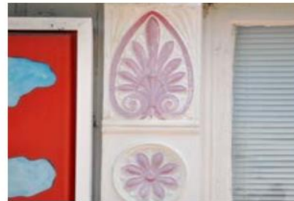
Detailing on Metal Pier
