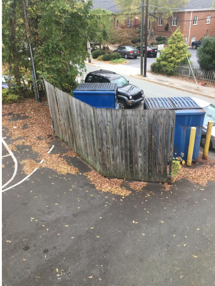
Existing fence (to be replaced) and trash dumpsters; Pickard Lane beyond
