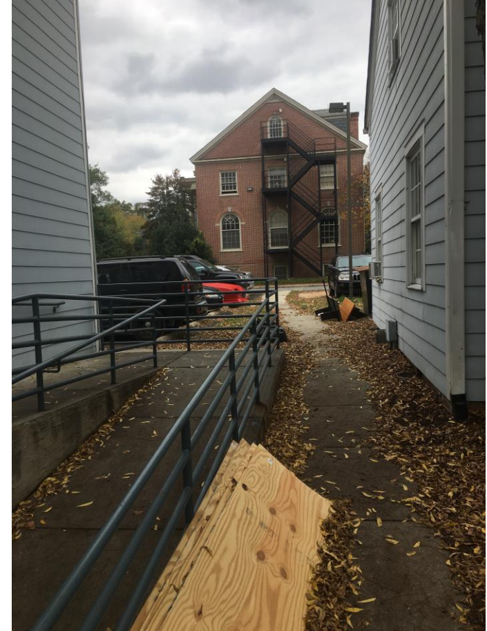
Facing West toward UNC Coates Building and site of proposed pedestrian gate
