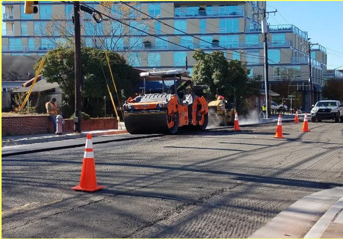
Street Resurfacing and Reconstruction
