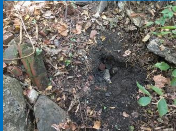
CCP Exposed At Surface
