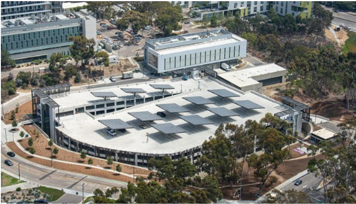
Photovoltaic (PV) Panels as “umbrellas” on roof
