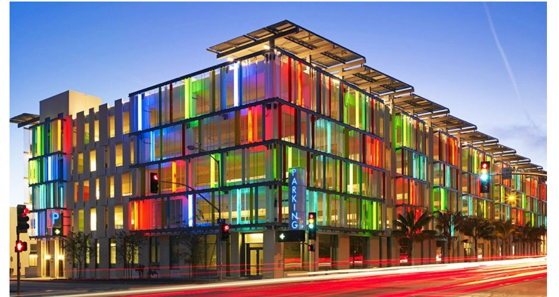
PV panels at edge of roof create a modern “cornice”
