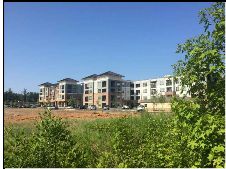
12 View of new construction to the south of the site.
