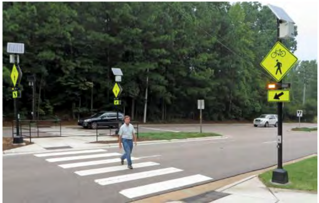
Example of rapid rectangular flashing beacons in Cary NC >
