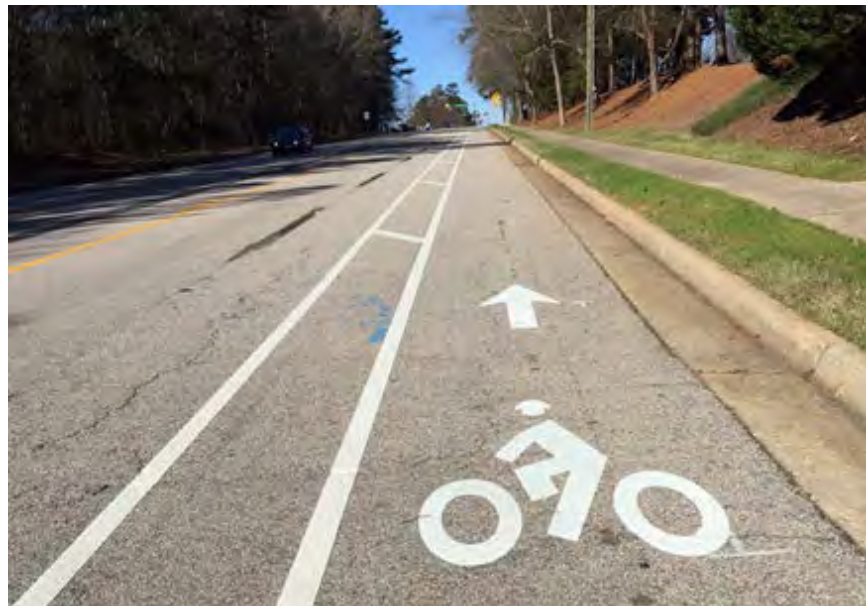
Example of a buffered bicycle lane in Raleigh >
