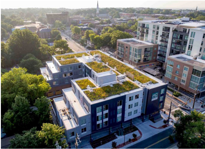
AC Hotel on Rosemary Street with green roof installed by Living Roofs, Inc.
