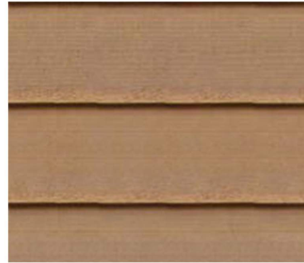
FIBER CEMENT CLADDING 1
