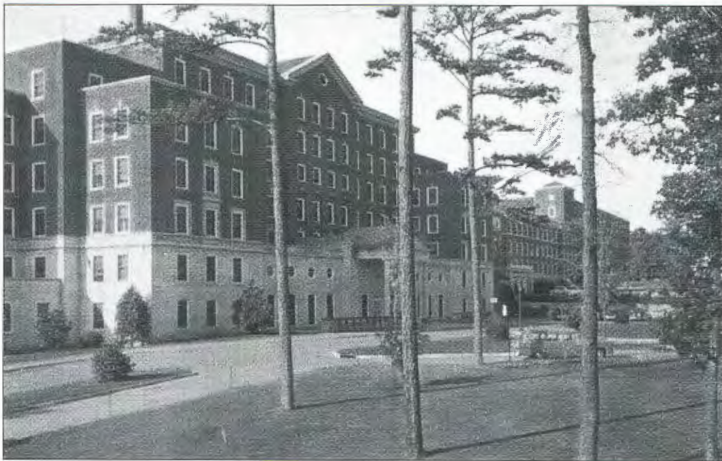
Figure 3. North Carolina Memorial Hospital, circa 1957
