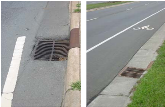
Left: sunken grate on Martin Luther King Jr. Boulevard marked with a diagonal warning stripe. Right: Level grate north of Homestead Road on Martin Luther King Jr. Boulevard
