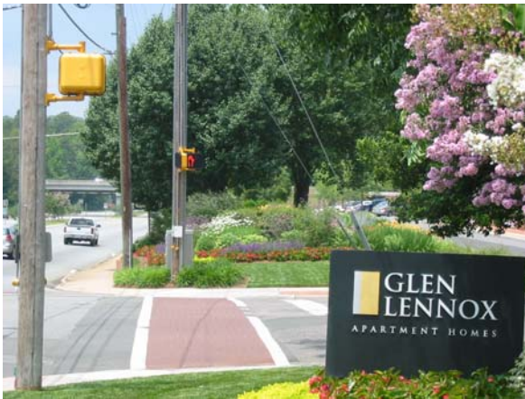
Photo: Existing crosswalk with push button activation and a colored / textured surface finish at Glen Lennox Apartments off NC 54
