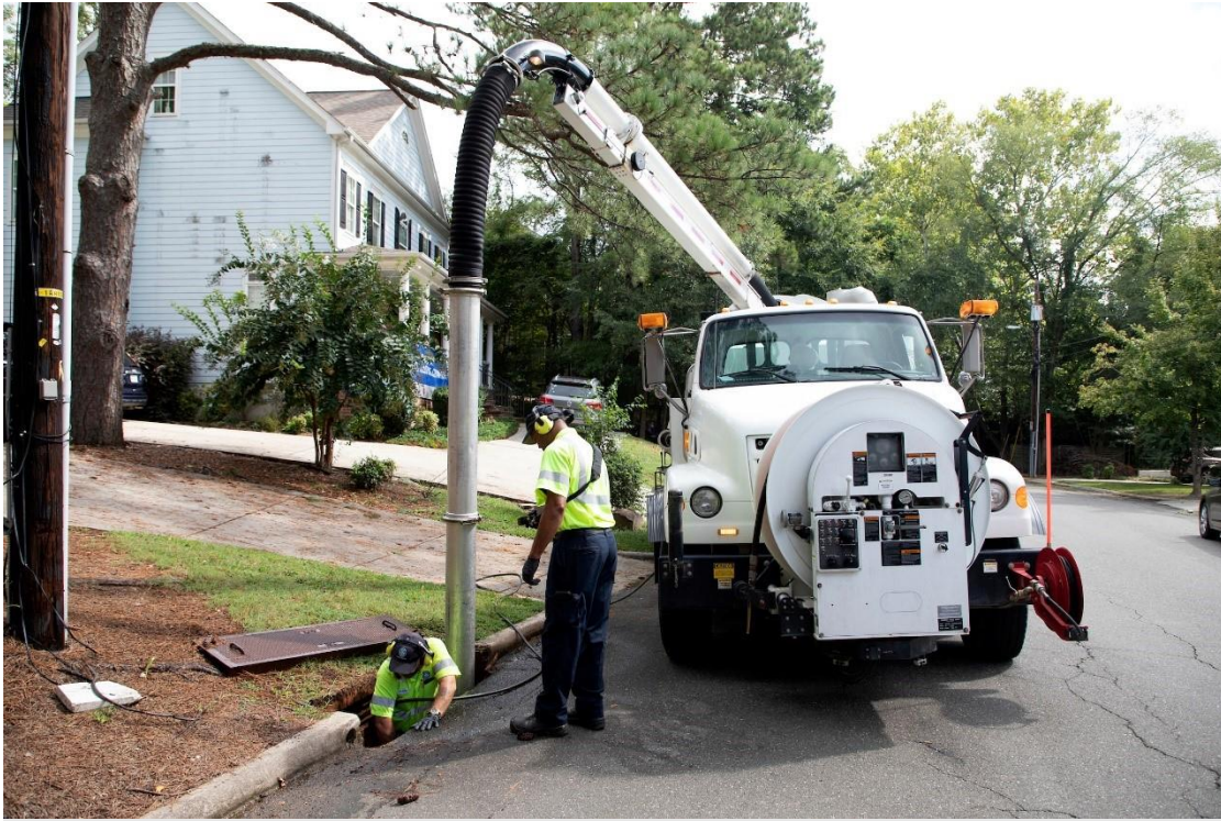
Stormwater maintenance crews clearing a storm drain
