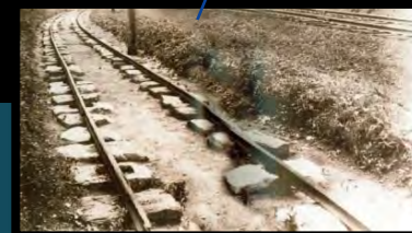
Trains & Iron Rails 170 years ago
