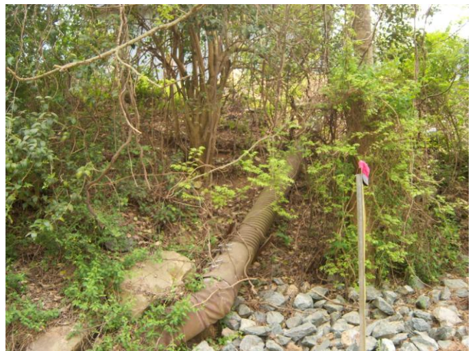
These photos show the ineffective pipe and some of the debris that once were buried in the bank, but are now exposed due to erosion. A longer term project will eventually address issues related to the bank and control of exotic plant species.
